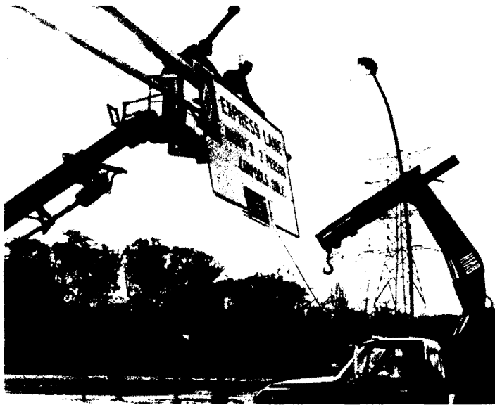
FIRST EXPRESS LANE SIGN — The first sign for the interim Express lane on Highway 12/Interstate-394 is lifted into place near the eastbound entrance west of Essex Road by State Highway Department employees.
