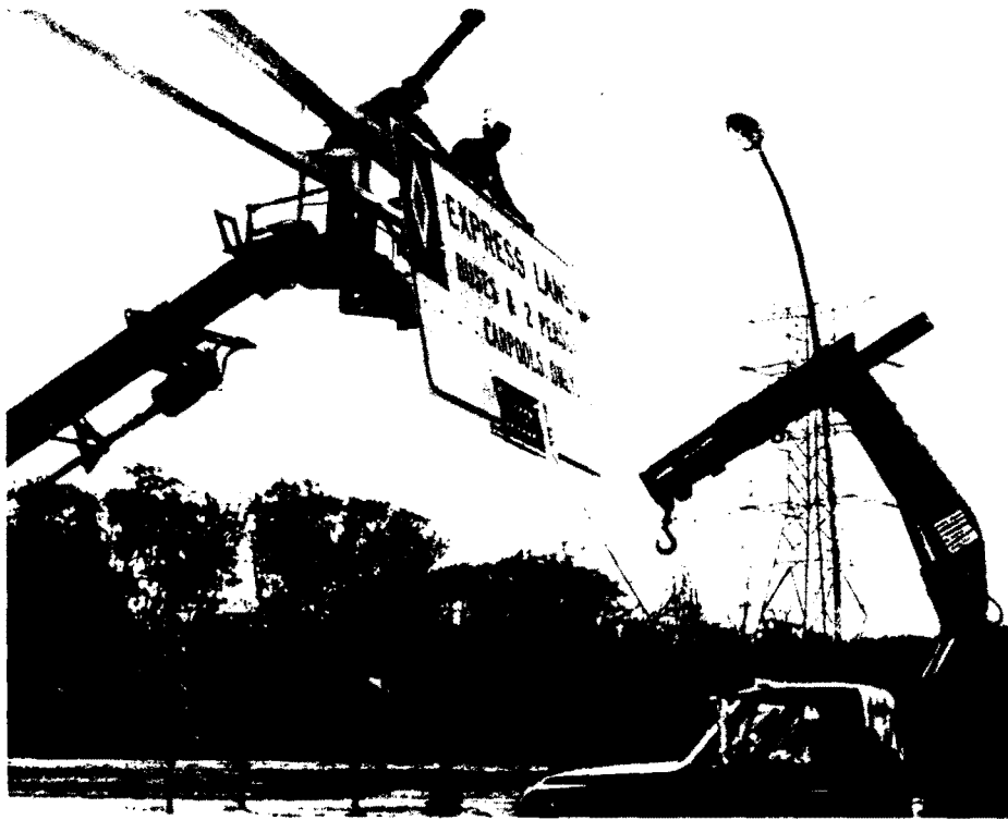
FIRST EXPRESS LANE SIGN —The first sign for the interim Express lane on Highway 12/Interstate-394 is lifted into place near the eastbound entrance west of Essex Road by State Highway Department employees.
