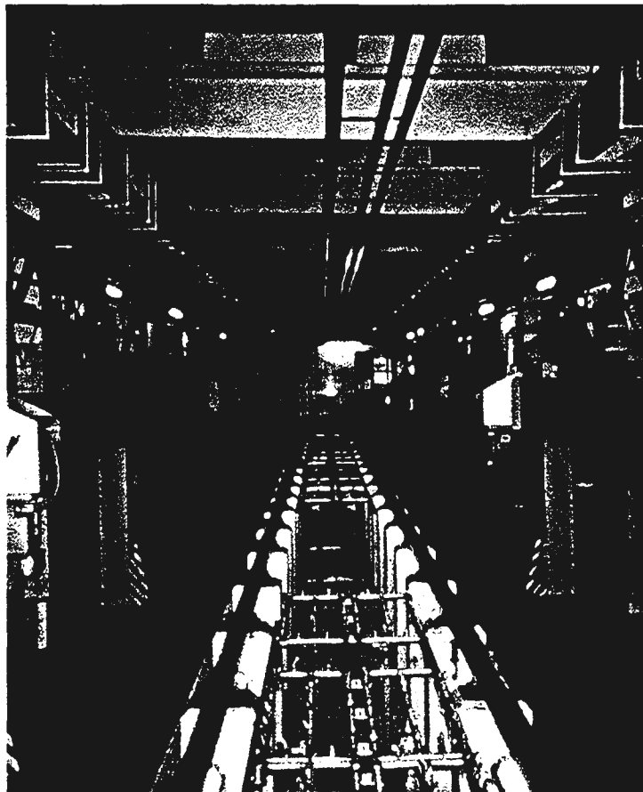
Figure 5.2.2/ Interior of Robotic Cleaning Bay
