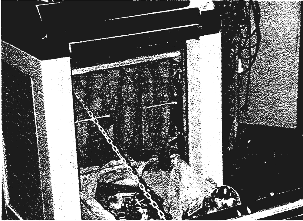
Figure 2.6.5.5/ C.A.B.X. Debris Collection Area with Fire Extinguishing System
