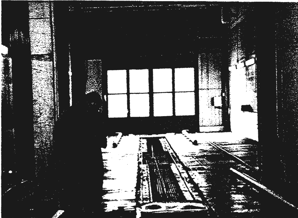
Figure 2.6.3.2.1/ Under Body Wash System
