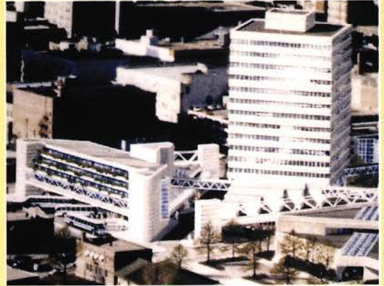
Ground Transportation Center Cedar Rapids, Iowa
