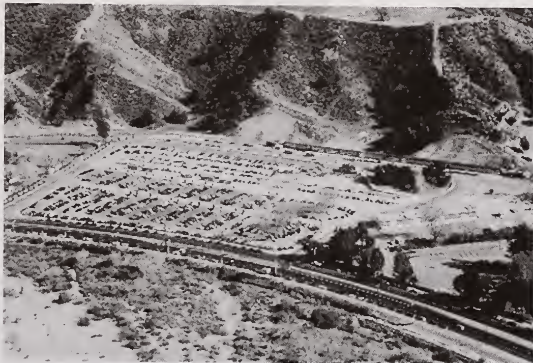
Shown here, the existing Santa Clarita Station with its parking lot at capacity.
