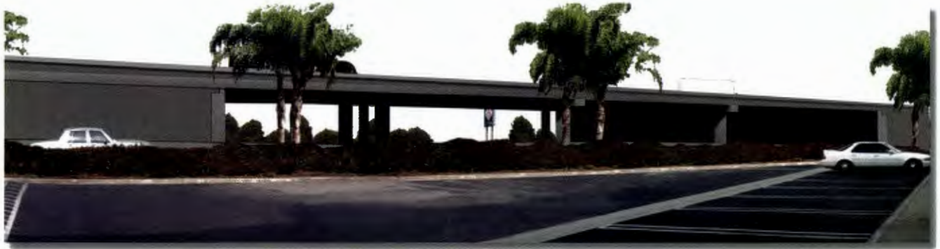
I-5 Interim HOV Improvements at Carmenita Road
