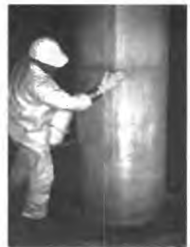
Pier concrete column after wrapping.
