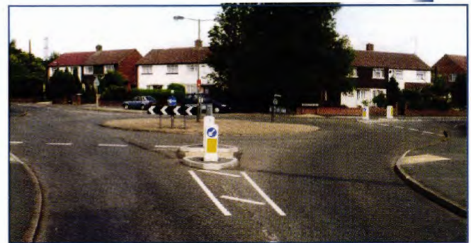
Figure 29. One-lane urban roundabout, England.
