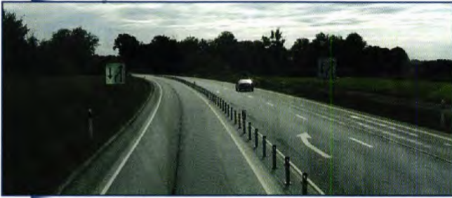
Figure 10. Use of cable barrier in 2+1 road, Sweden.
