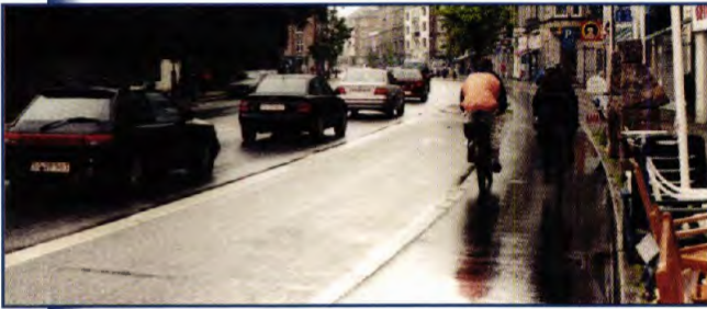
Figure 36. Bike path elevated and separated from roadway, Denmark.
