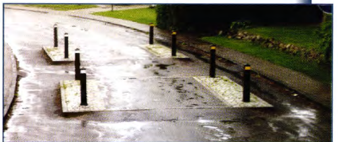
Figure 17. Narrowing with humps, Denmark.
