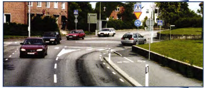
Figure 22. Small roundabout flush with pavement, Sweden.
