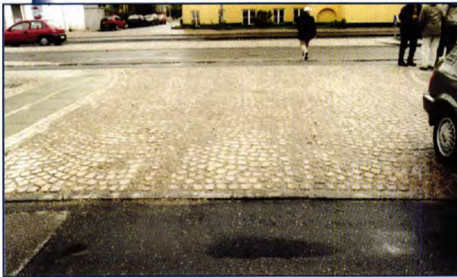
Figure 27. Table with different pavement texture, Denmark.
