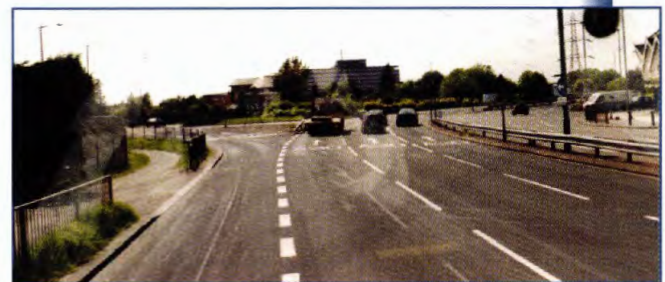
Figure 30. Roundabout with three lanes and traffic signal control, England.
