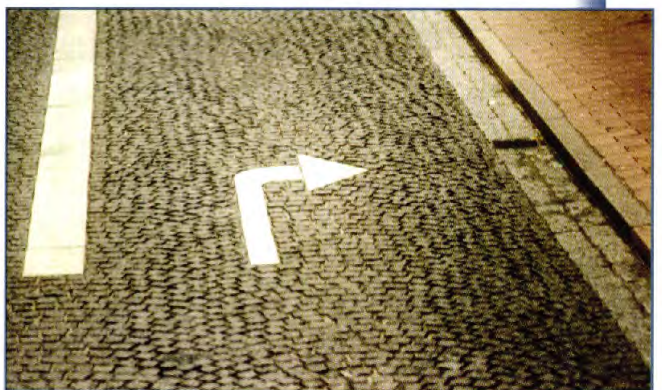
Figure 25. Lane markings as part of pavement texture, Denmark.
