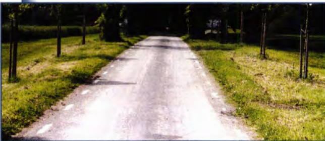
Figure 13. Optical narrowing by eliminating centerline, Sweden.
