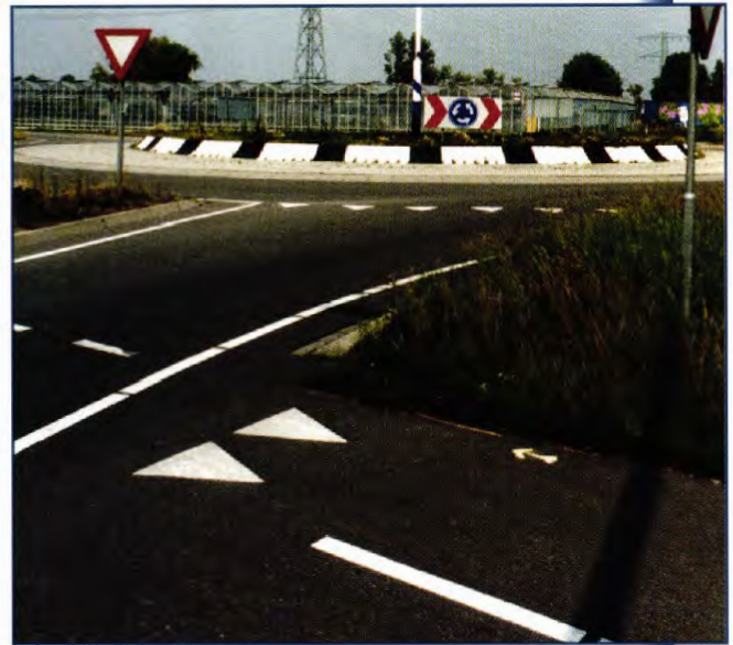
Figure 28. One-lane rural roundabout with bike lane, The Netherlands.
