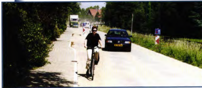
Figure 19. Narrowing by eliminating one lane, The Netherlands.
