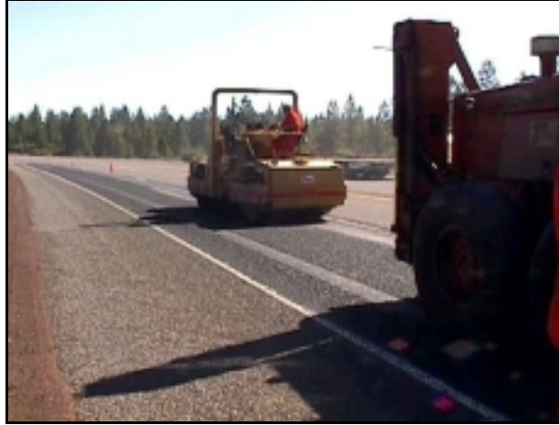
Figure 4.37: Compaction with Steel-Wheeled Roller
