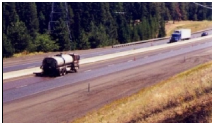
Figure 4.1: Fog Sealing EB Passing Lane, I-84 near MP 239.9, July 1997
