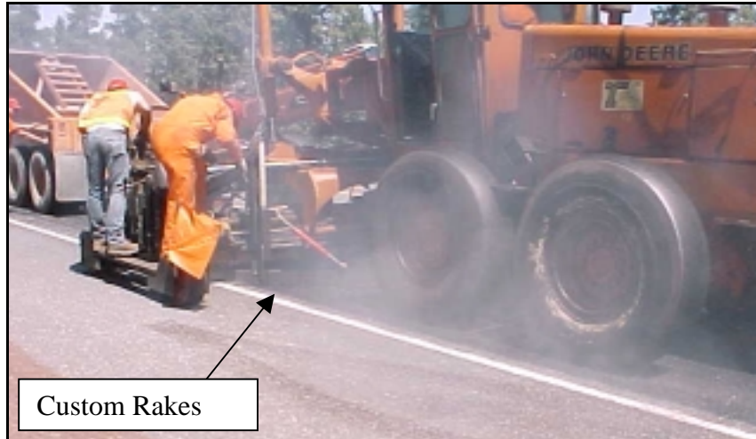
Figure 4.35: ODOT's "Barber Orange"
