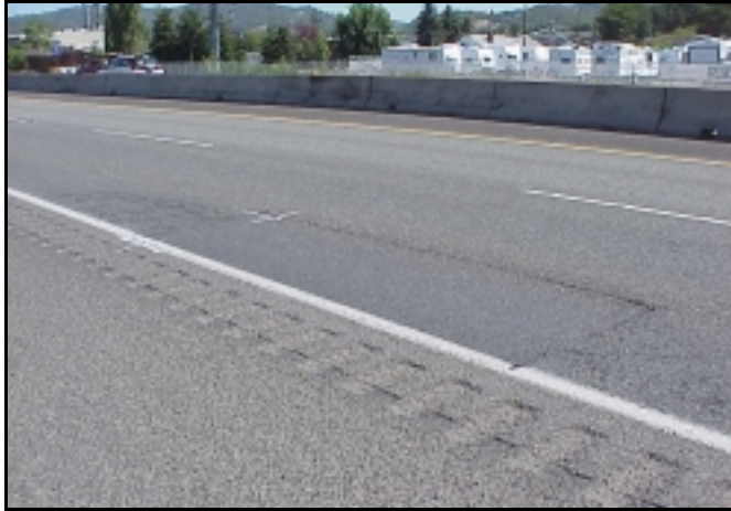
Figure 4.28: Plug Patch on I-5 SB in Roseburg
