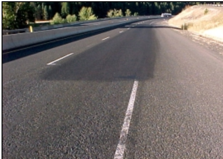
Figure 4.7: Blade Patch near MP 253.2 WB, September 2001
