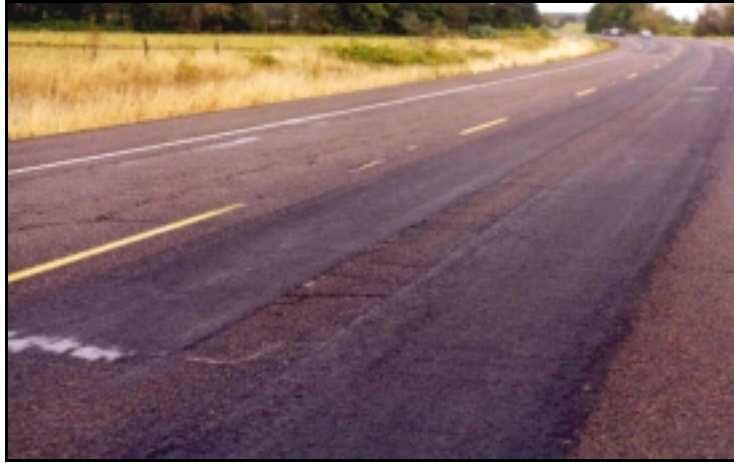
Figure 4.17: Close-up of Newly Placed Screed Patches, 1997
