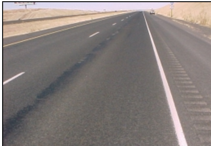
Figure 3.17: Stripping Looking West, September 2001
