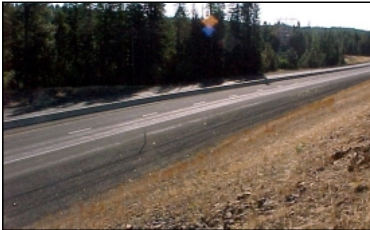
Figure 4.2: EB Lanes (foreground), I-84 near MP 239.9, September 2001
