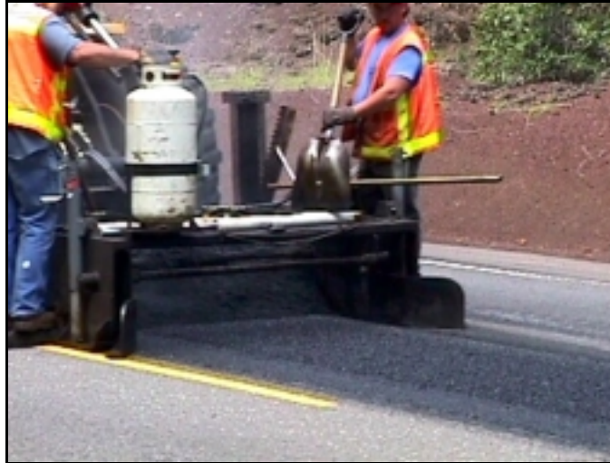
Figure 4.22: Close-up View of Screed Box and Windrow
