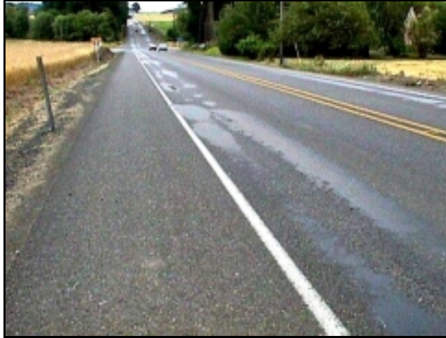
Figure 3.12: ORE 99W Looking South to McCoy Junction
