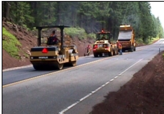
Figure 4.20: Screed Patch Procedure Viewed from Behind the Equipment
