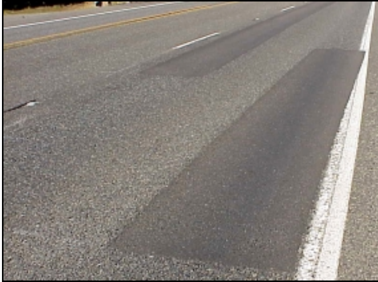
Figure 4.31: Successful Plug Patch on ORE 42 near MP 58 EB, 2001
