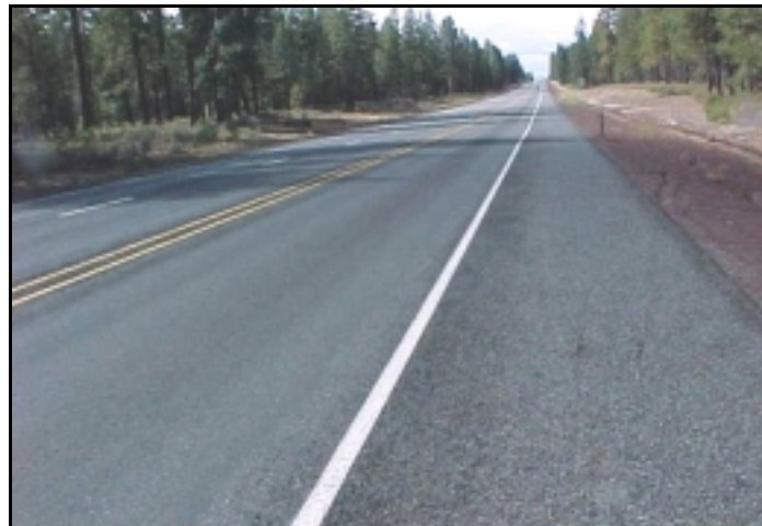
Figure 4.34: Repair of Nearby Stud Rutted Area after Two Years of Traffic
