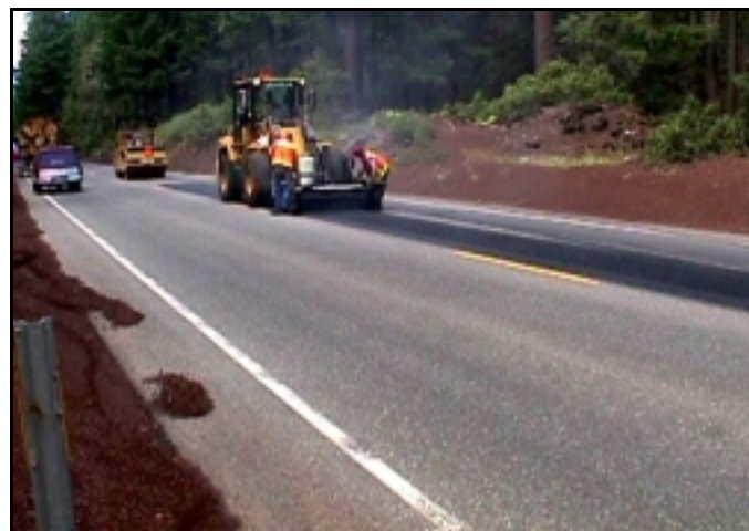
Figure 4.21: Front View of Screed Box and Windrow
