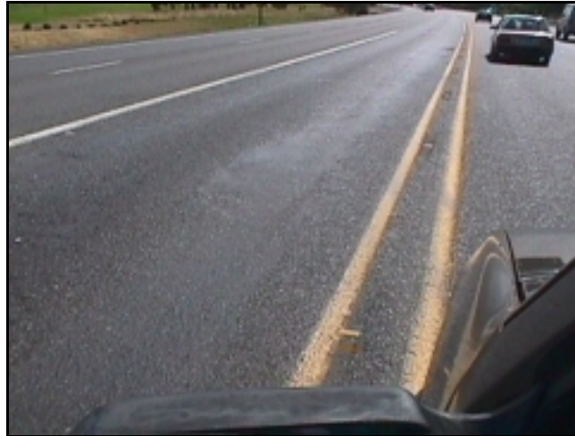
Figure 3.5: Deformation Rutting in WB Left Turn Lane from ORE 34 to Corvallis Bypass, August 5, 1999
