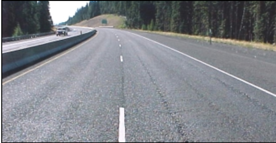
Figure 4.5: Same Location as Figure 4.5, Four Years after Fog Seal, September 2001.
