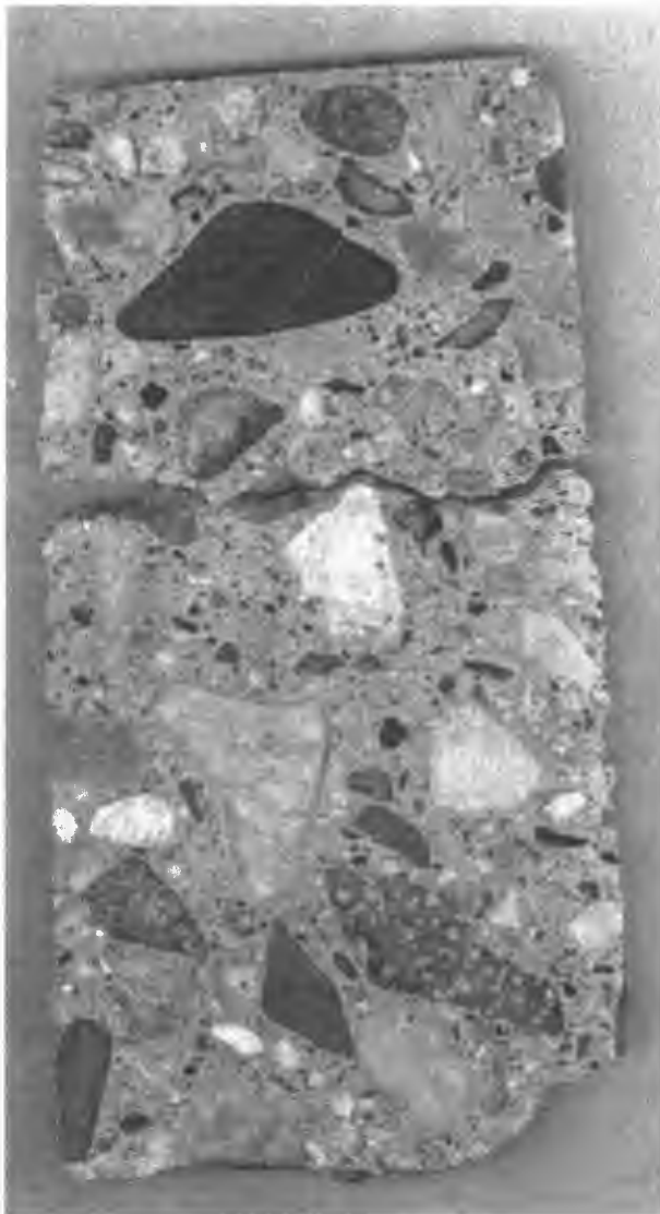
(a) Stained slab
