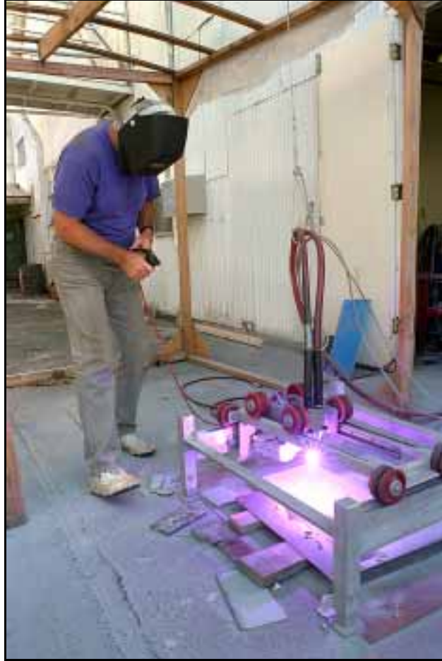
Figure 4.1: Thermal-spraying of zinc onto new slabs with robotic-controlled x-y passes
