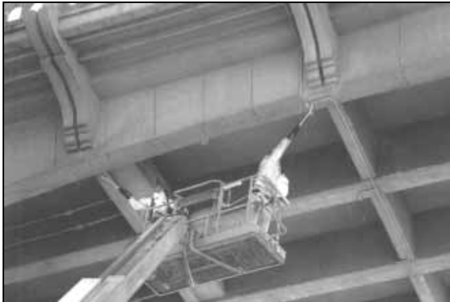
Figure 4.5: Application of humectants under the deck of the Yaquina Bay Bridge
