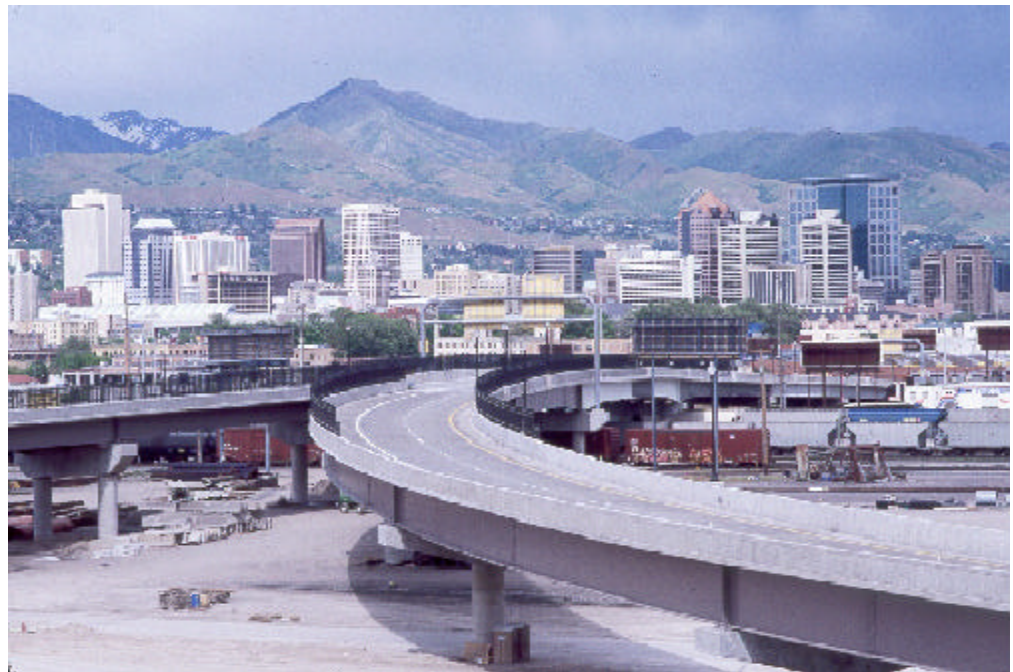
Design-build contracting combines project design with construction to save time and allow greater flexibility on complex highway projects, like this multi-lane expansion on I-15 in Utah.
