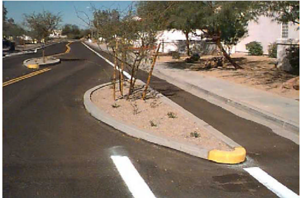
Traffic calming and context-sensitive design techniques in Phoenix, such as lane narrowing and bicycle lanes, use the roadway itself to reduce traffic speeds instead of police enforcement.
