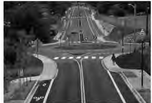
The addition of bicycle lanes and sidewalks create space for pedestrians, while medians and landscaping narrow the street width and slow traffic.
