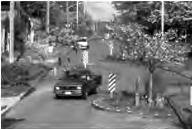
The chicanes pictured above narrow this residential street to one lane and require traffic to move slowly.
