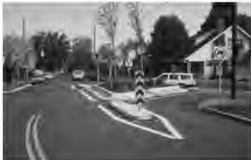
Traffic diverters restrict certain traffic movements and should only be considered when less restrictive measures are not appropriate.
