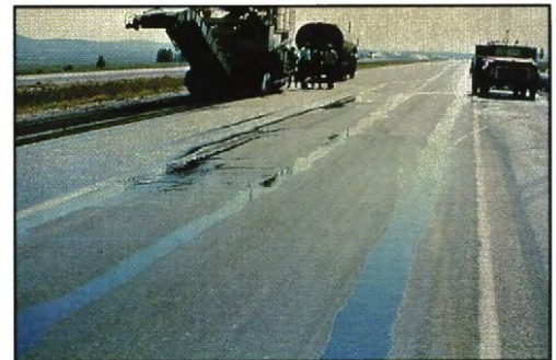
FIGURE 33 Distress Type ACP 9—Standing Water in Ruts
