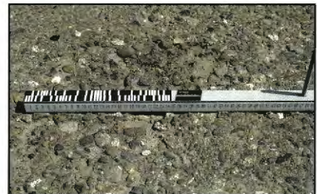
FIGURE 42 Distress Type ACP 13—Loss of Coarse Aggregate
