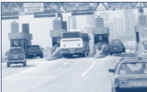
Toll roads are the major means of providing new road infrastructure in Latin America.
