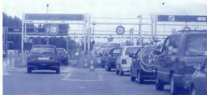
Figure 11. Drivers who use France's Télépéage electronic tolling system can pass through tollbooths without stopping. (Courtesy Association Des Sociétés Francaises D'Autoroutes)
