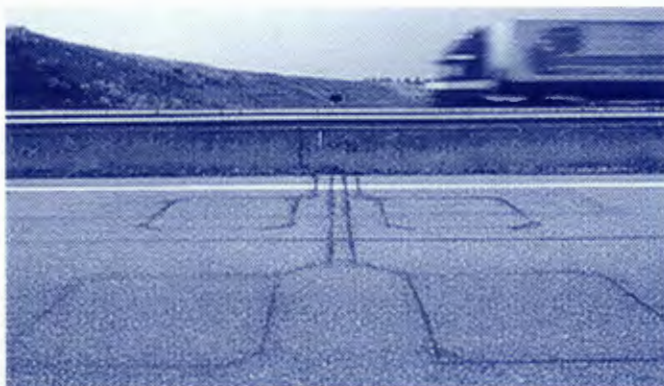
Figure 9. Detection loops in the road surface yield data for use in traffic congestion monitoring and incident response. (Courtesy Policy Document on Traveller Information, The Netherlands)
