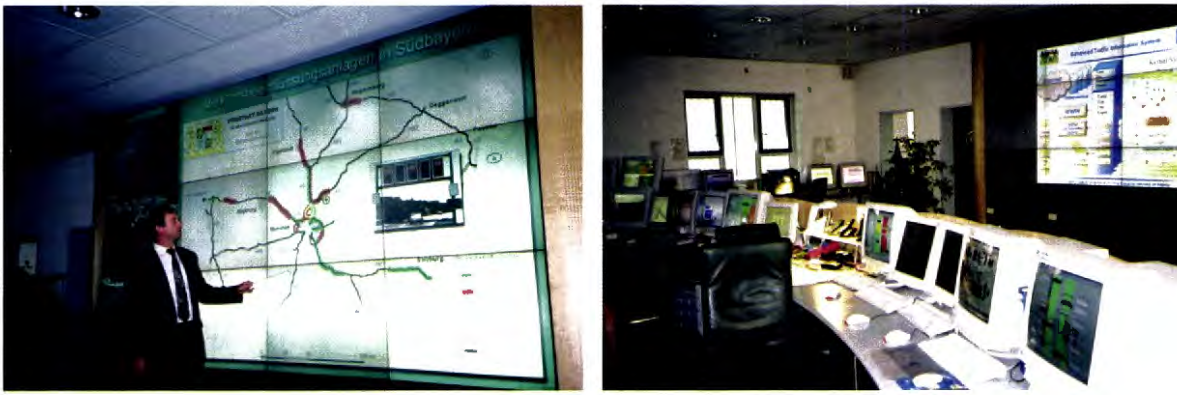
Figure 27. VRZ traffic management center.
