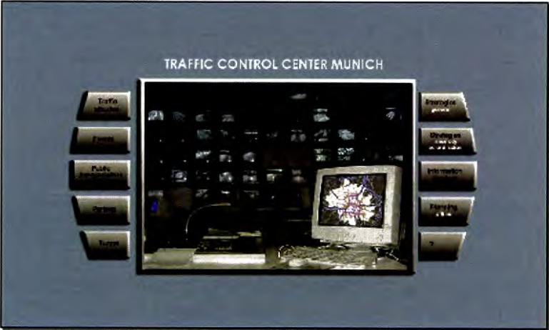
Figure 24. Traffic control center, Munich.
