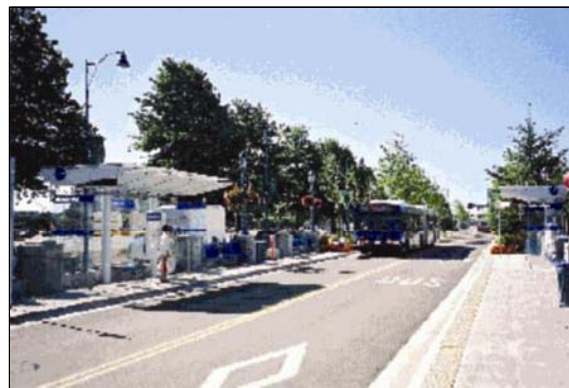
Station – Platform Layouts - Extended Platform with Un-Assigned Berths Vancouver 98-B Line Station
