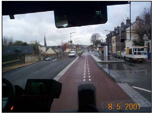
Running Way – Guidance View through Windshield following Optical Guidance Markers
