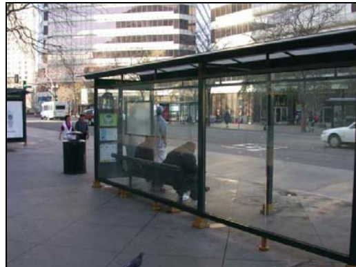
Station – Off-the-shelf station shelter in Oakland, CA
