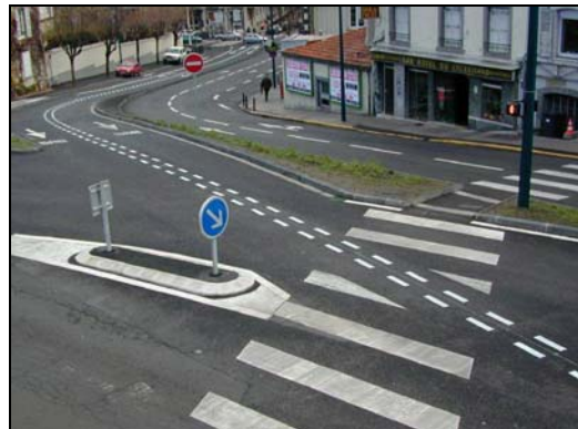
Running Way – Guidance Optical Guidance Markers in Rouen France
