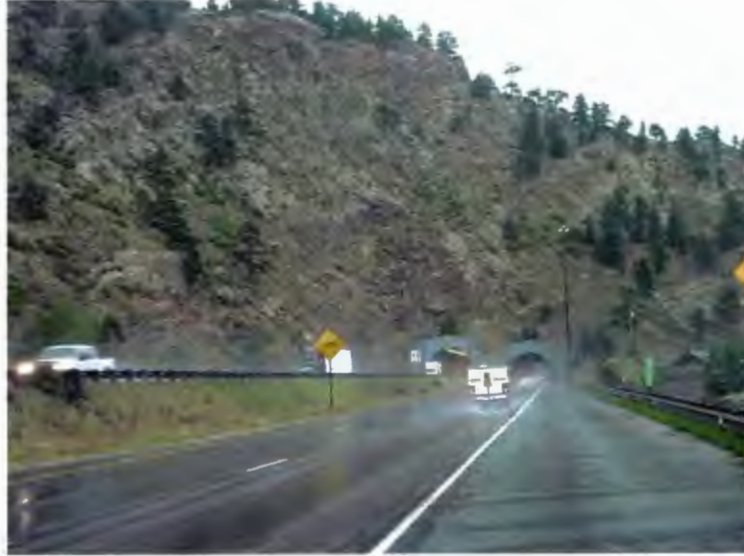
Figure 17: I-70 Eastbound at Twin Tunnels
