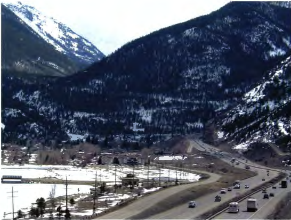
Figure 98: Photograph of I-70 looking westbound at Georgetown Lake
