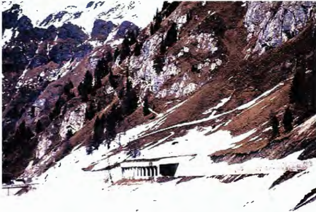
Figure A.1.2: Avalanche shed located in the Swiss Alps.
