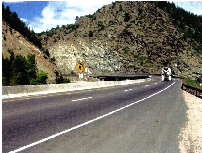
Figure 16: I-70 Westbound at base of Floyd Hill
