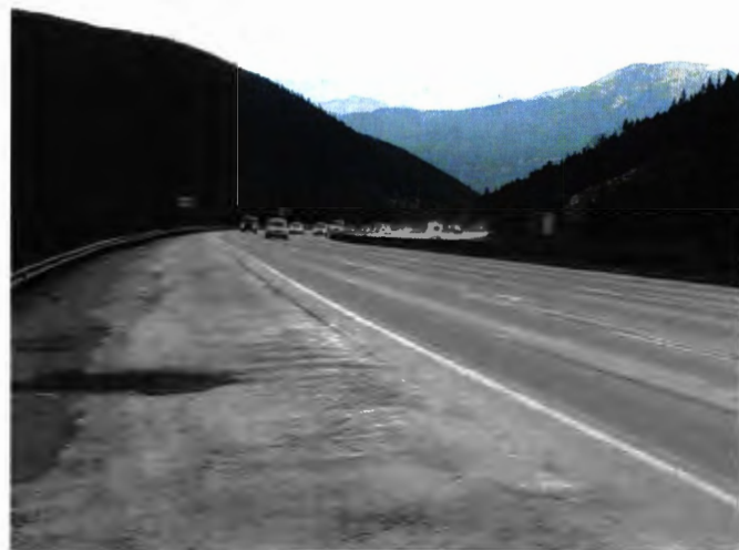
Figure 21: I-70 Westbound west of Eisenhower-Johnson Memorial Tunnel
