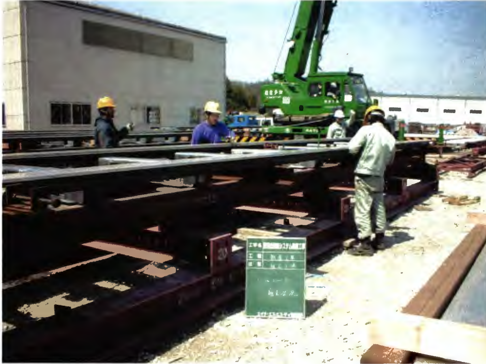
Figure 46: Levitation Rail Section Assembly Prior to Installation
