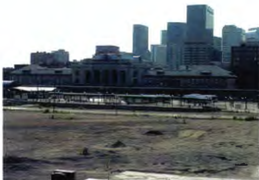
Figure 3: Denver Union Terminal
