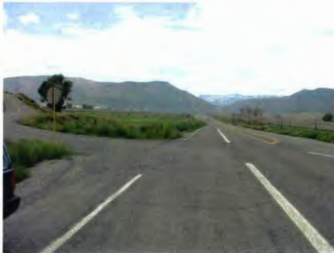
Figure 25: Eagle County Airport access roadway
