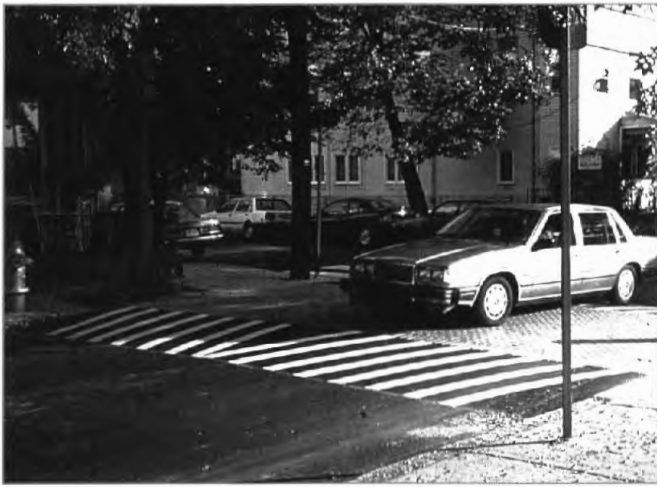
Raised crosswalk at Berkshire and Hardwick.
