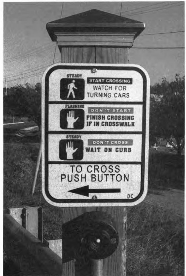
Example of an pedestrian regulatory sign used in conjunction with a pushbutton. The recommended language for such signs can be found in Section 2B.44 of the MUTCD.
