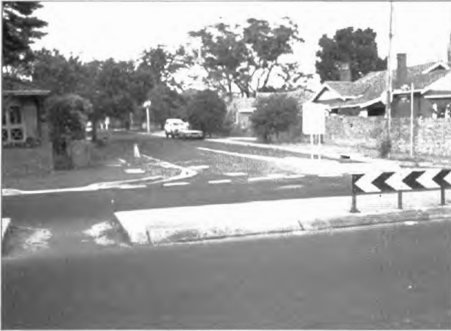
Intersection median barriers need to keep walking and bicycling flowing freely through the neighborhood.
