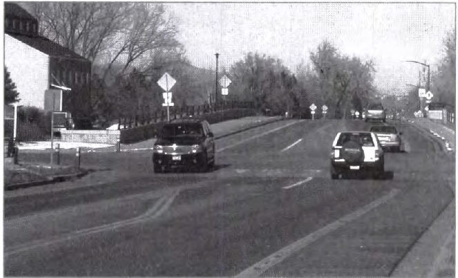
Second Raised Crossing on 55th Street.
