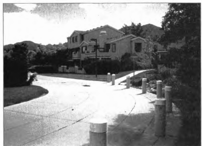
The curves in Walden Circle were designed to slow vehicles traveling through the Bridgewalk development.
