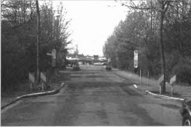
This choker narrows the street from two lanes to one. Traffic is forced to slow down and, in some cases, wait for an approaching vehicle to pass before proceeding.
