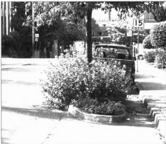
Mid-block landscaped bulb-out with parallel parking.
