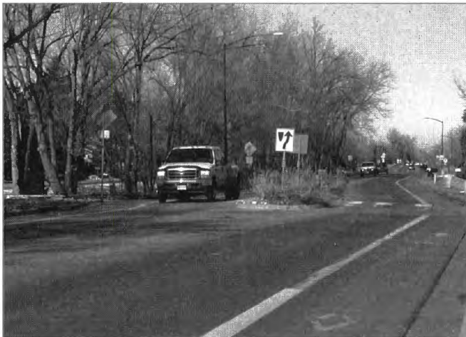
New concrete raised crossing with pedestrian refuge median on 55th Street.
