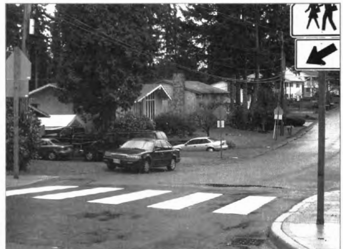
A raised crosswalk and curb extension along a street in the Bennett Elementary School Area.
