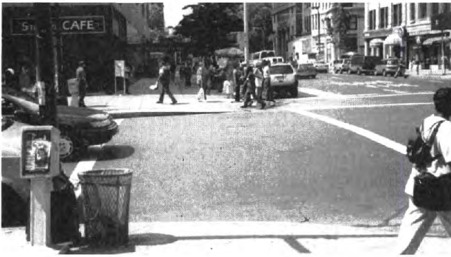
Standard Parallel Line Crosswalk
