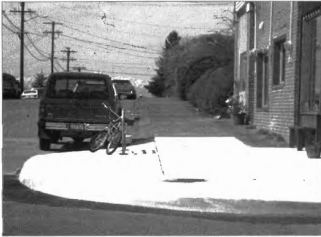
A curb extension on a residential street in Seattle, Washington. In addition to improving pedestrian safety at this intersection, the extension provides additional sidewalk space for a bicycle rack and accessible curb ramp.
