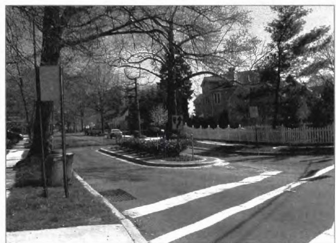
Gateway island at intersection.
