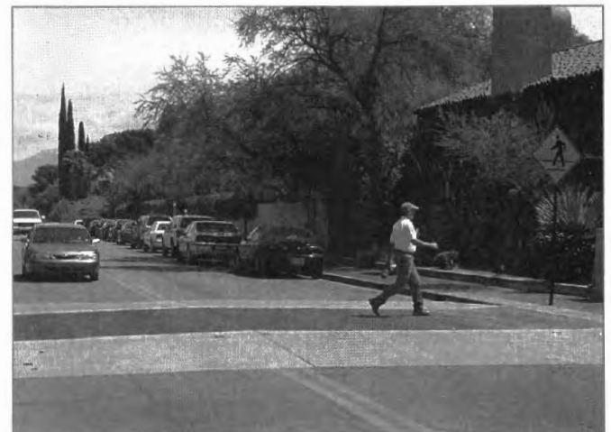
The slight slope and contrasting brick design of the raised crosswalk indicates the designated space for pedestrian crossing to approaching motorists.
