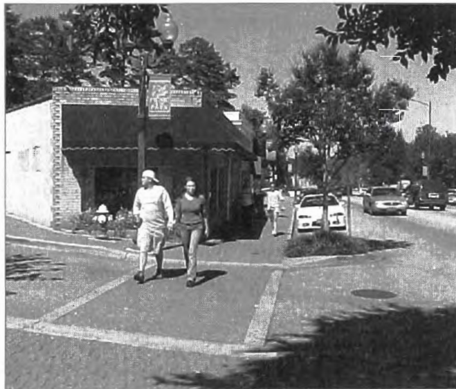
Pedestrian enhancements on College Avenue at Sloan Street include brick pavers, curb ramps, and new landscaping.
