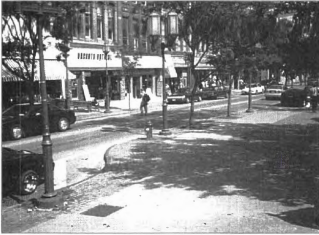
A mid-block curb extension on Main Street in Oneonta, NY narrows the street to two lanes and cuts the pedestrian crossing distance in half.
