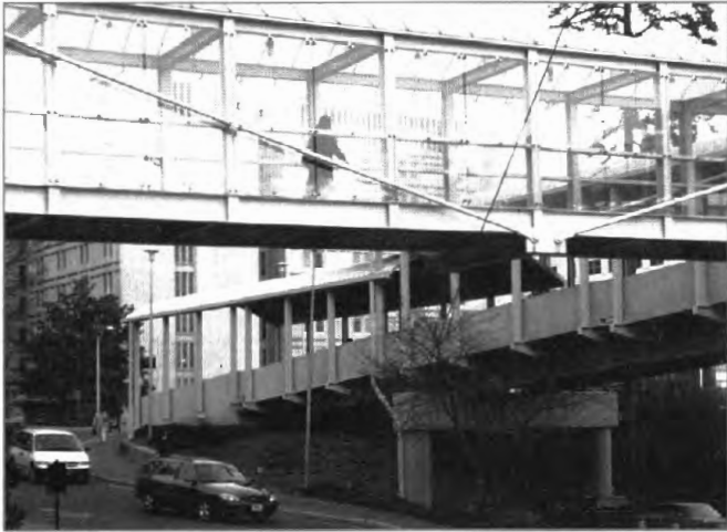
This pedestrian overpass takes advantage of existing topography and allows pedestrians to avoid conflicts with traffic at street level.
