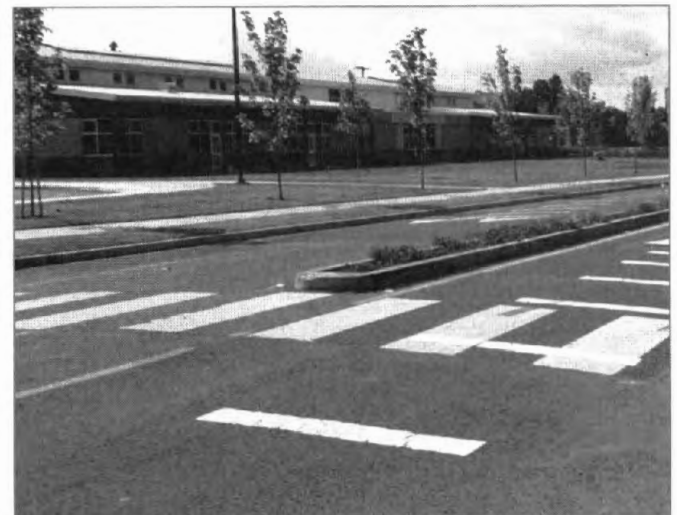
View of the emergency response speed hump on the east end of the project.
