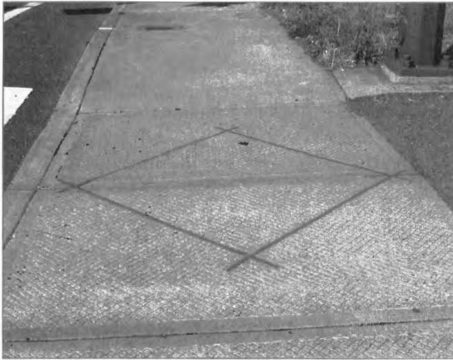
A bicycle-activated Signal Loop Detector.
