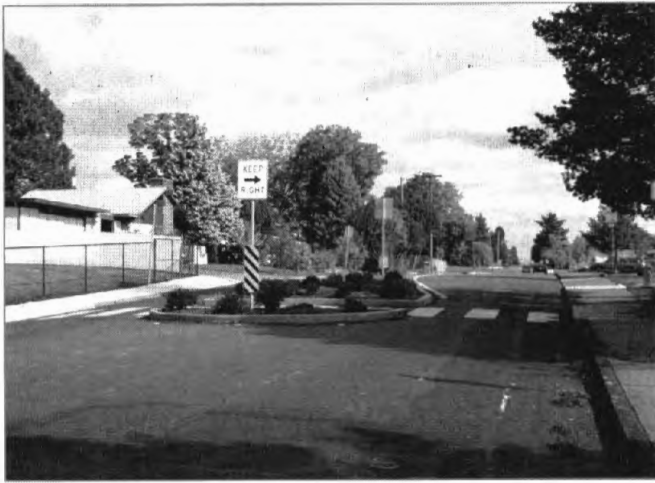
View of the median slow point with pedestrian crossing in the center of the median.
