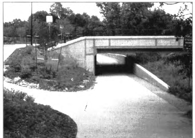
New bicycle/pedestrian underpass beneath 55th Street.
