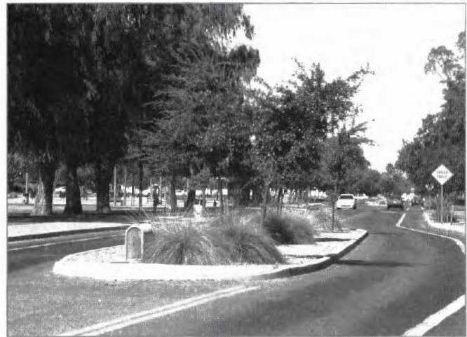
A median island and bicycle lanes encourage slow vehicle speeds and wide sidewalks provide pedestrian access along Fifth Street.
