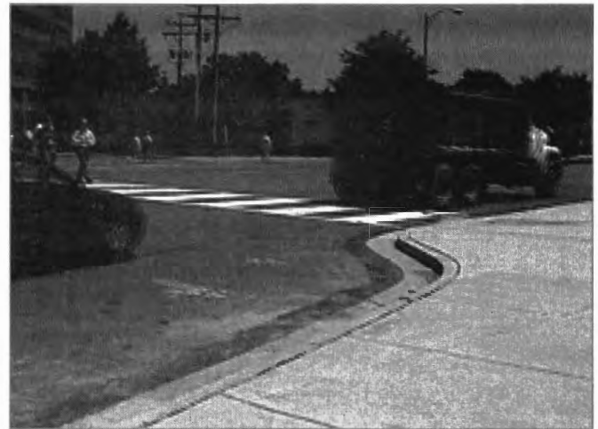
Curb extension and crosswalk on Wilson Boulevard.
