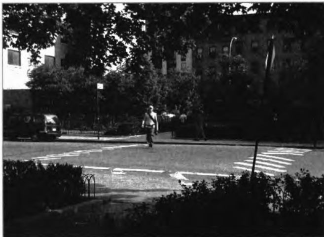
Pedestrians use the speed table as a raised crosswalk.
