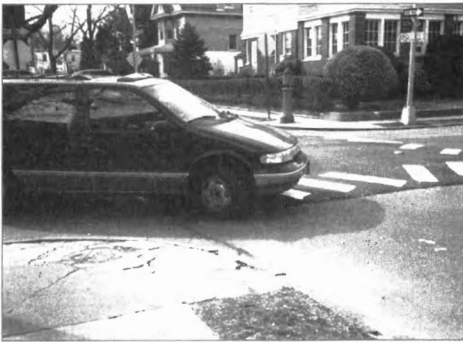
Turning vehicles must round the corner with one set of wheels on the hump.
