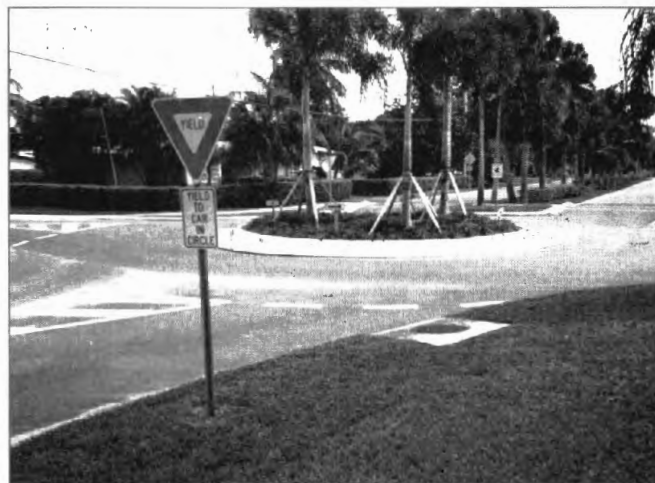
Median island and intersection roundabouts were installed on 7th Avenue.
