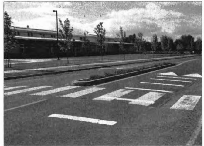
An emergency response speed hump.
