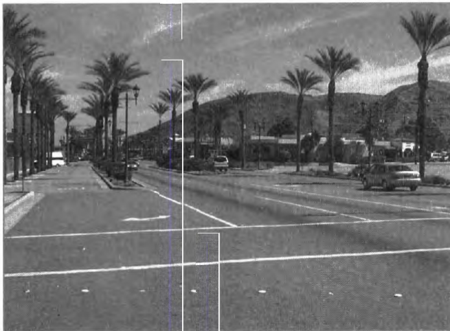
Looking east showing the use of protected/separated right turn and bus lanes.
