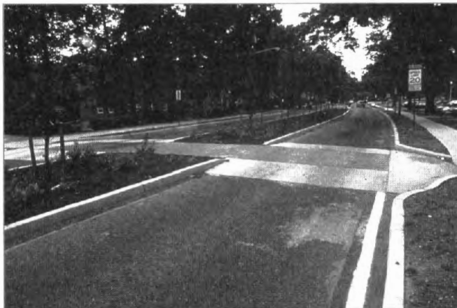
A raised pedestrian crossing provides a continuous route for the pedestrian at the same level as the sidewalk. Pavement markings may be used on the slope to make the crossing visible to motorists.
