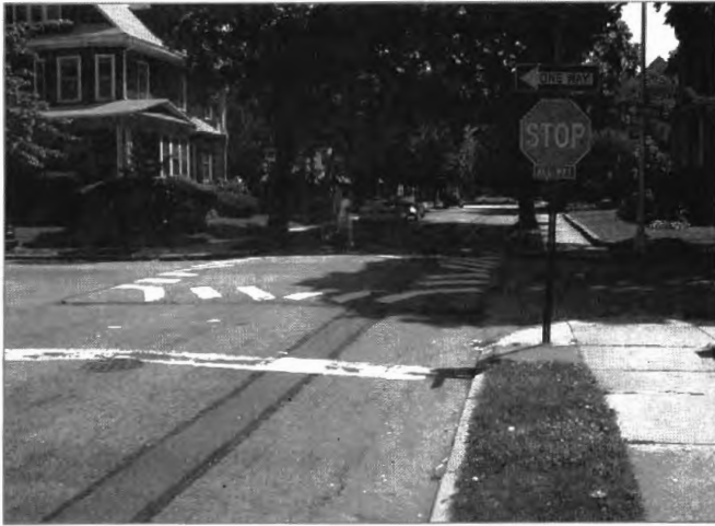
The raised intersection reinforces the all-way stop.
