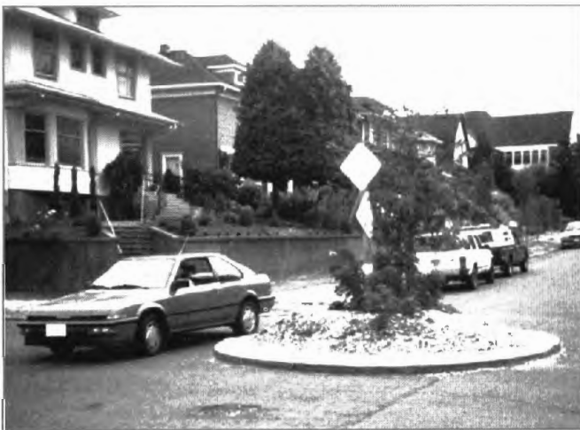
A traffic mini-circle helps reduce vehicle speeds, but still allows cars and emergency vehicles to pass through the intersection with little difficulty.
