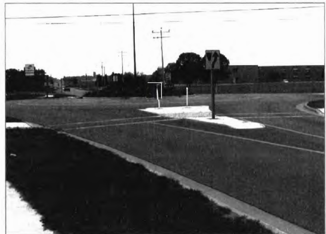
An approach to one of the modern roundabouts near the Howard school campus.
