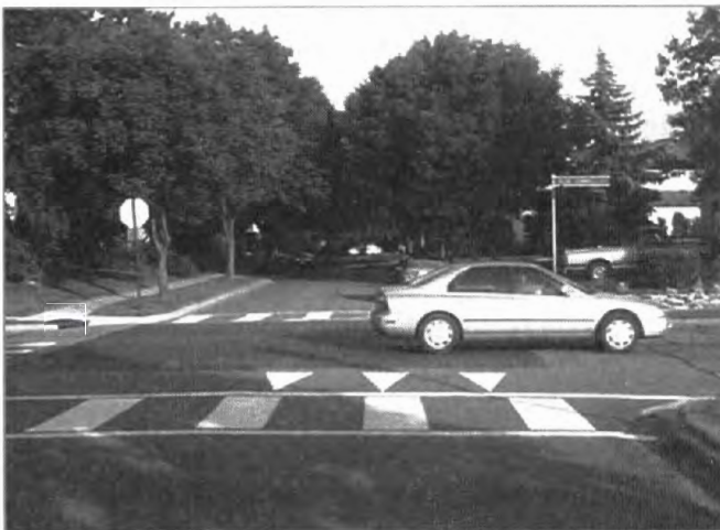
A raised intersection slows all vehicular movements through the intersection and improves pedestrian crossings in all directions.
