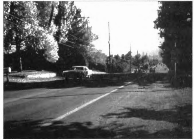
First Street was a two-lane road with no curb, gutter, or sidewalks before it was improved.
