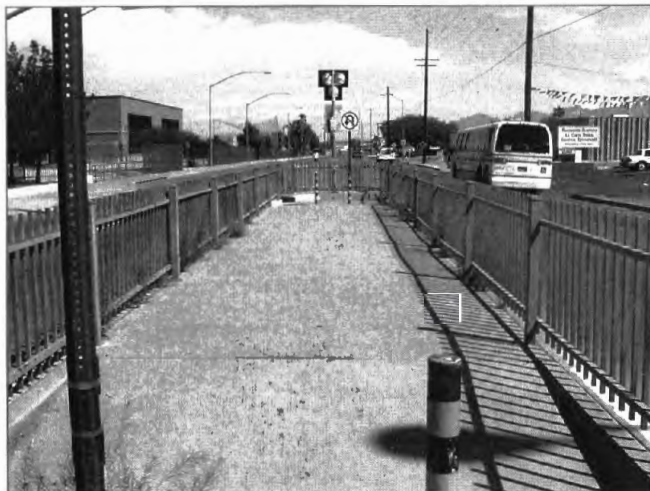
Close-up of fenced pedestrian refuge median.
