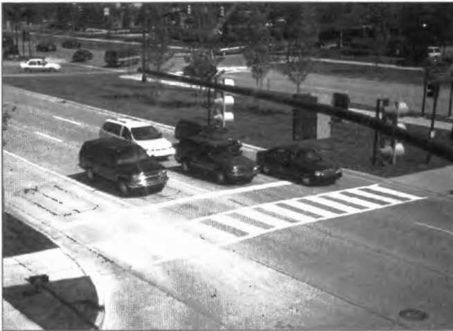
The “ladder” pattern shown above is more visible to motorists than parallel lines and requires less maintenance if painted to allow the tires of motor vehicles to track between the painted lines.
