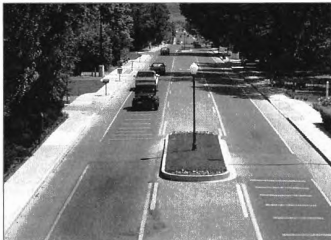
Medians, speed tables, and raised crosswalks have been effective at reducing vehicle speeds.
