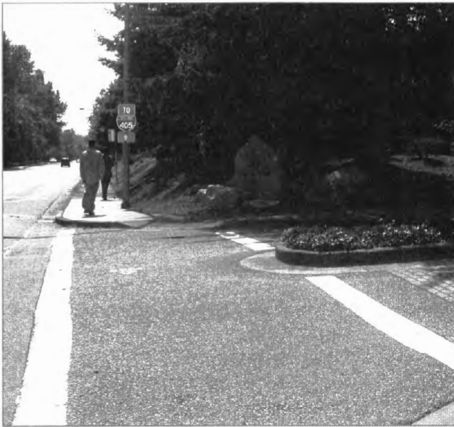
A landscaped island with pavement treatments at the entrance to the Surrey Downs neighborhood.
