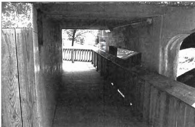
The extensive use of wood made the structure strong, practical, inexpensive, and aesthetically pleasing.
