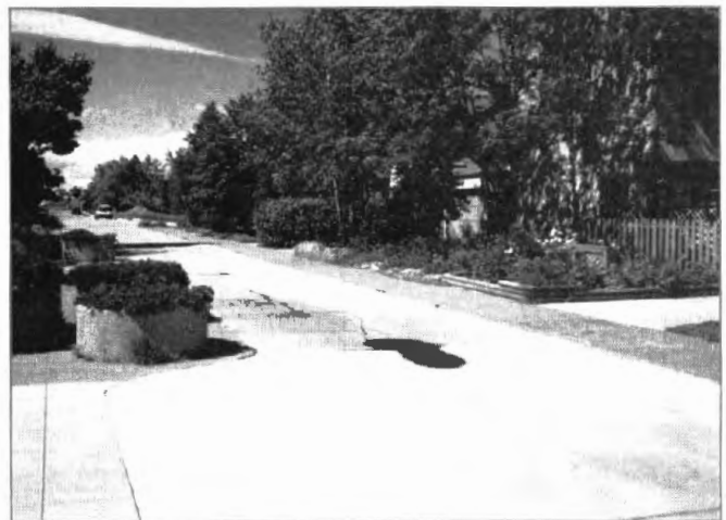
The narrow street and landscaping of The Cottages development encourage slow vehicle speeds.
