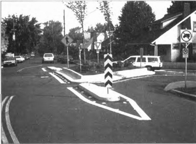
This modified T-intersection in Portland, Oregon, is intended to reduce speeds of through traffic as well as restrict left-turning vehicles.
