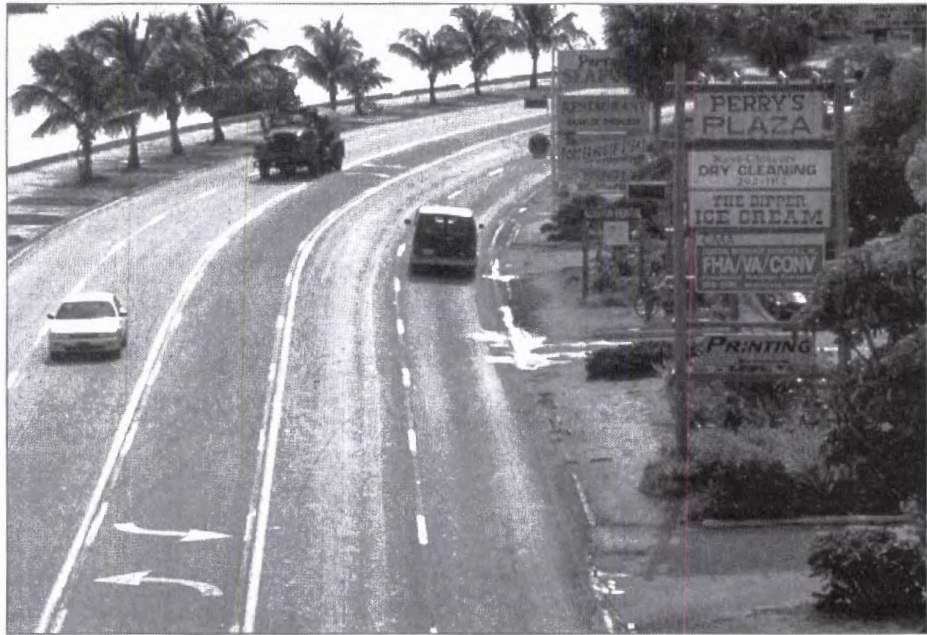
This roadway may act as a barrier to pedestrians. Those who are walking along the waterfront may find it difficult to cross to the commercial establishments and those on the commercial side may be reluctant to cross to the waterfront.
