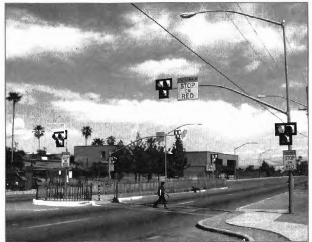
Staggered median with HAWK beacon (MUTCD experimental device) at bus stop.
