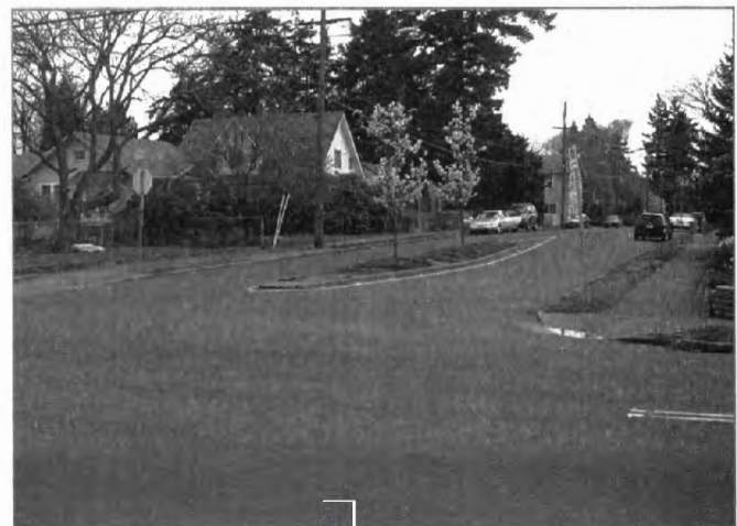
The median island on Harold east of 52nd Avenue slows turning vehicles.
