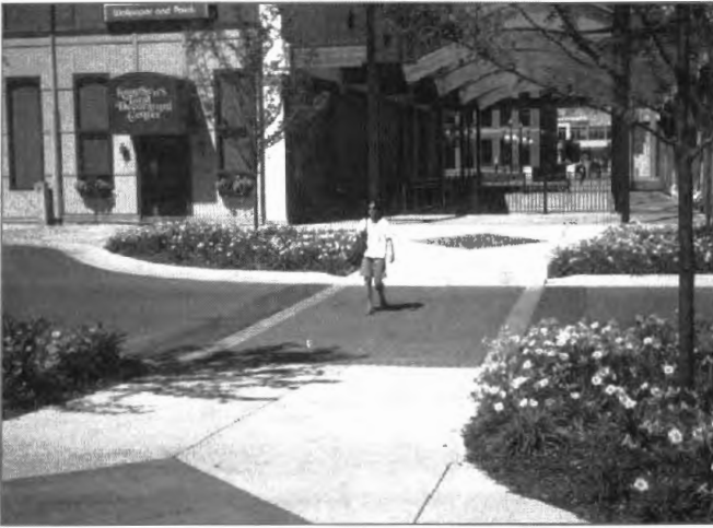
This midblock crossing is in Kalamazoo, Michigan. The landscaping and textured crosswalk are visually appealing and provide a clear message about where pedestrians can be expected to cross the street.
