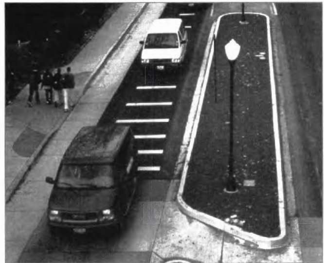
The sidewalks, raised medians, and raised crosswalks on First Street accommodate pedestrians effectively.
