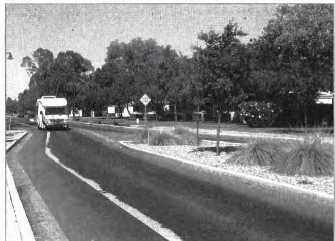
A median island and bicycle lanes encourage slow vehicle speeds and wide sidewalks provide pedestrian access along Fifth Street.
