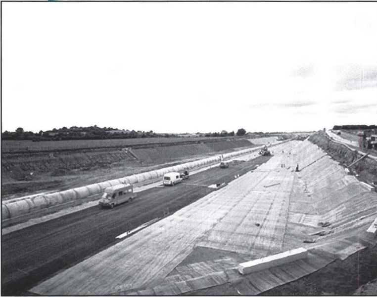
Figure 5. Demonstration of bituminous membrane application in Denmark. (Photo source: Colas Danmark A/S, Denmark)
