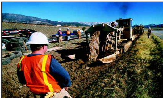
Figure 8-1: Fiber Cable Route Construction – Photograph Courtesy Adesta, LLC
