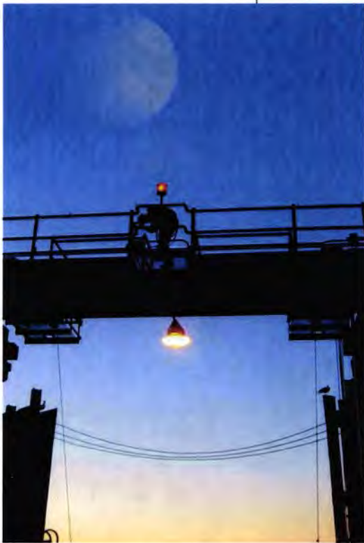
Fig 6 – Antenna installation on terminal
