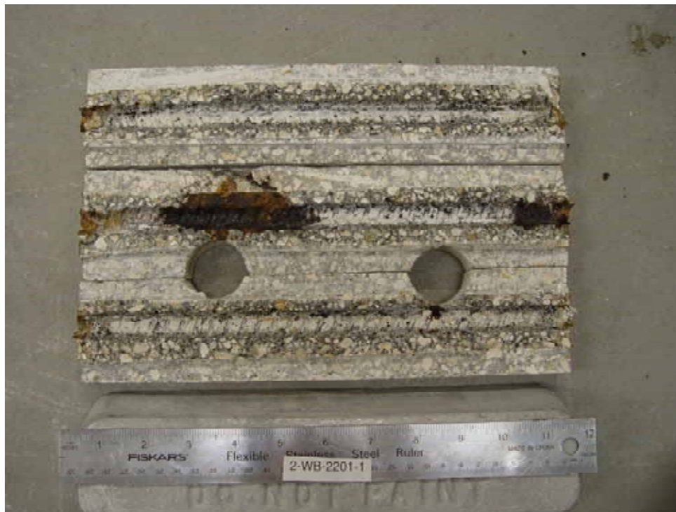
Figure 4.107. Photo. Trace of the upper rebars and corrosion products on specimen number 1-WB-2201-1.
