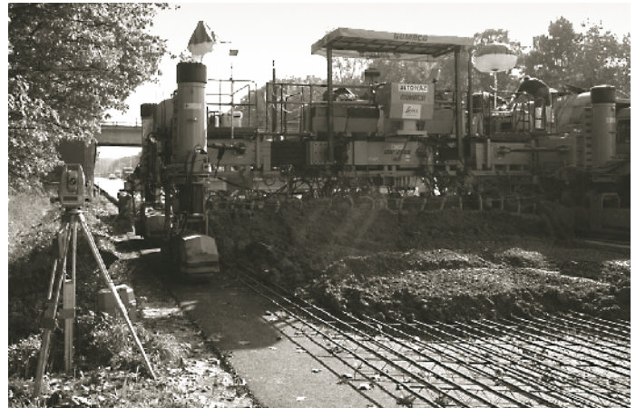
Figure 45. CRC overlay paving on E40/A10 in Belgium.
