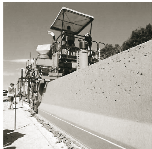
Figure 46. Slipform paving of the safety barriers on the E40/A10 CRC overlay project.
