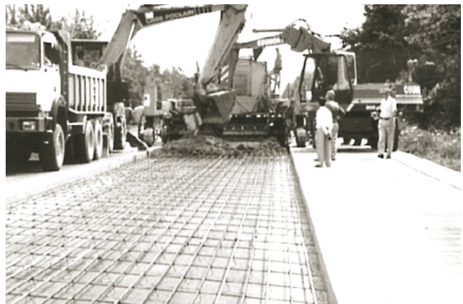
Figure 41. CRC inlay construction in Belgium.
