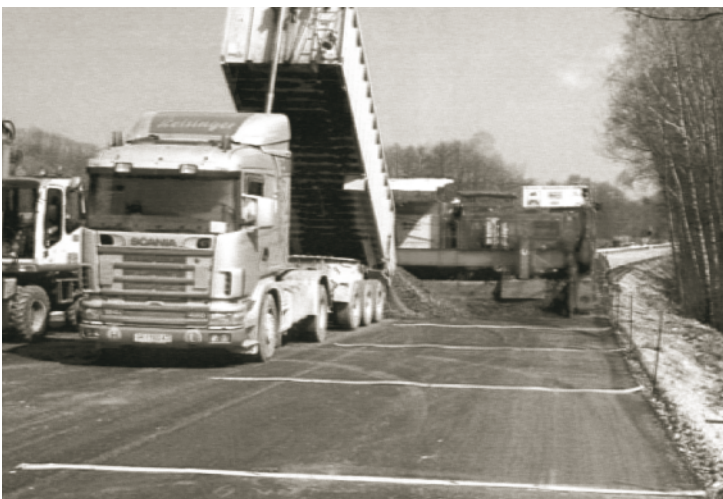
Figure 32. Flat drain tapes placed before paving.
