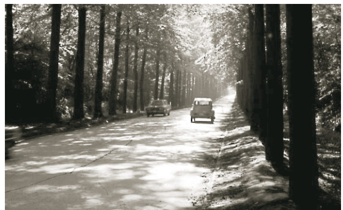
Figure 12. Belgium's first concrete pavement, built in 1925, remained in service for 78 years.
