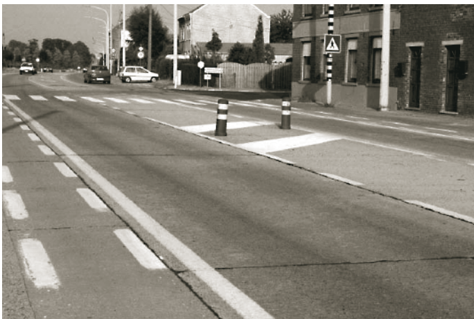
Figure 42. Belgium's first concrete overlay after 45 years in service.
