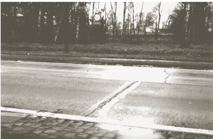
Figure 25. Concrete pavement in Belgium still in service after 55 years.
