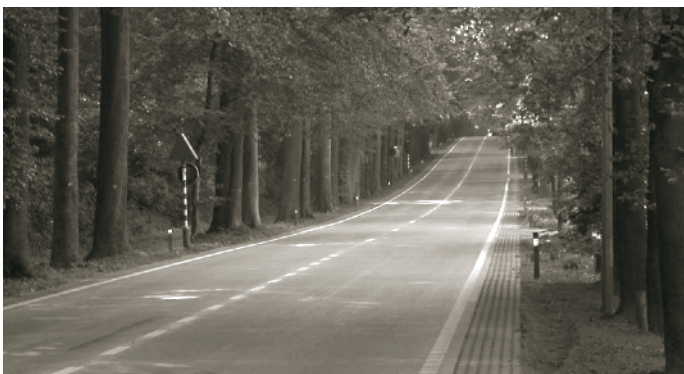
Figure 43. Concrete overlay constructed in 2003 on Avenue de Lorraine in Brussels.
