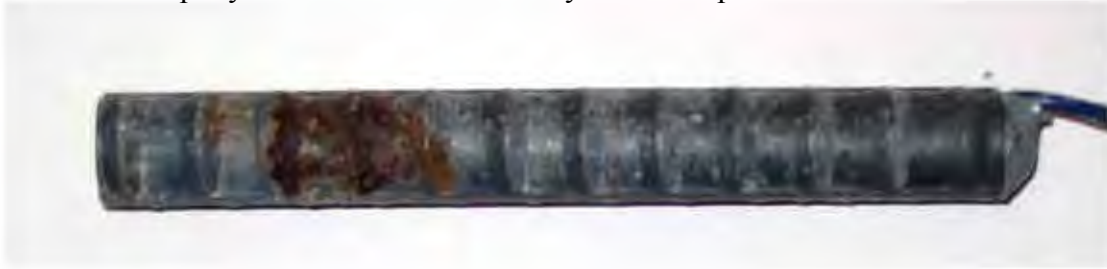
Figure 17. Photo. Conventional anode bar after removal of mortar, at 15 weeks.
