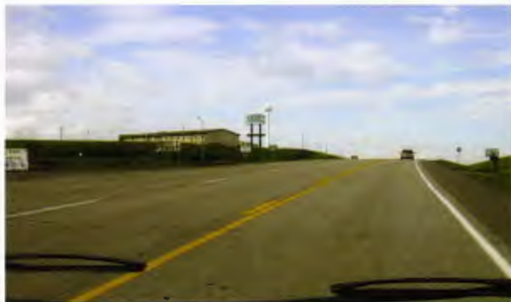
US 12 at Grand River Casino (left), near Mobridge, SD
