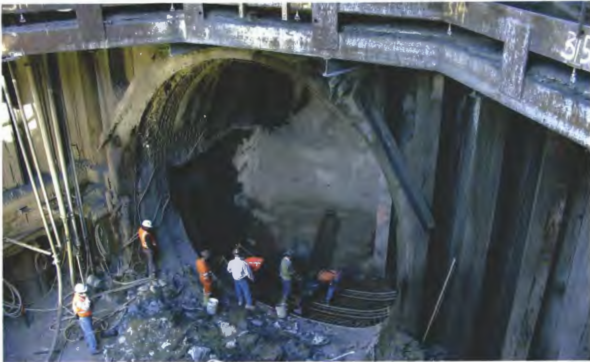
Figure 3-1: Excavations for Silver Line tunnel at Russia Wharf (MBTA)
