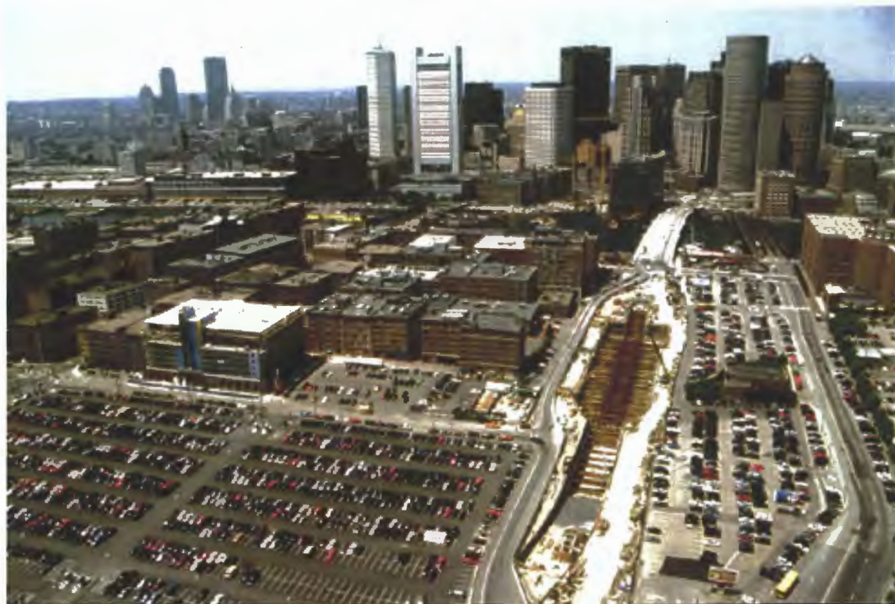
Figure 3-3: Aerial view of Silver Line construction (MBTA)
