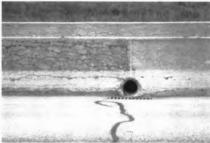
Figure 15. Barrier wall in Quebec—the section of the wall to the right of the picture has been treated with a silane sealer.
