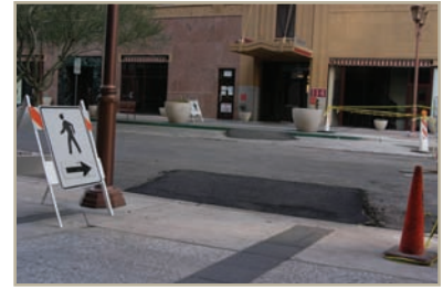
A stable, temporary curb ramp
