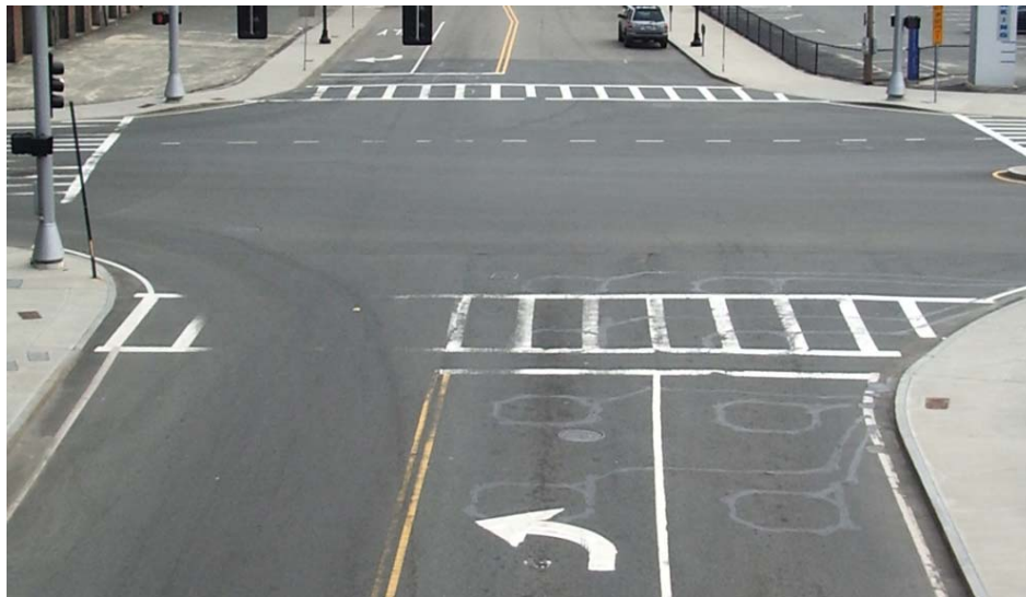
(b) Physical representation of loop detectors
