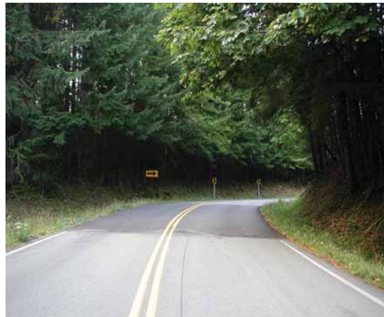
View of a curve along Lewis River Road with existing curve warning signs.
