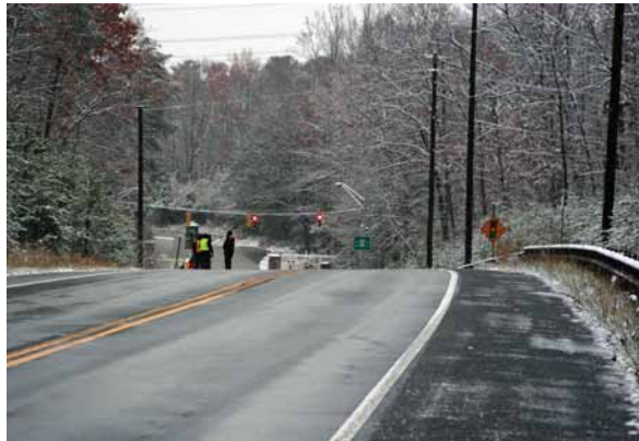
SIGNALIZED INTERSECTION OF POWDER MILL ROAD AT MD 197, MD
