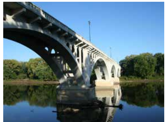
Historic Indiana bridge: Knox. Photos courtesy of Indiana DOT.
