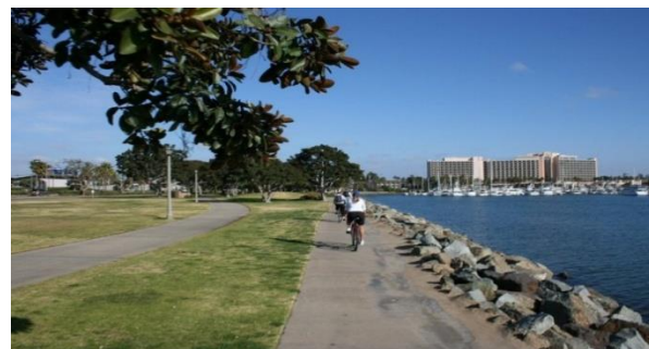
Figure 3: Bikeway (Concrete Bicycle Path)
