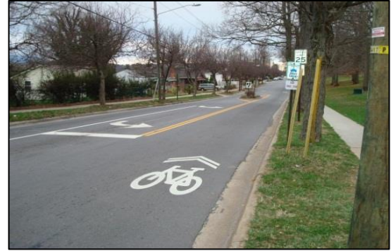
Figure 32: Shared Lane Marking
