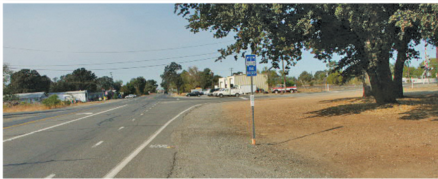
Left: The lack of an accessible path makes it difficult for a person using a wheelchair to access this stop in Red Bluff, California. All patrons would have to travel on gravel and on the roadway shoulder to use the stop. Source: G. Araki.
