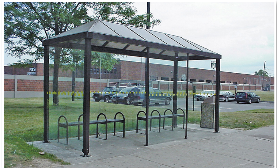
This shelter in Rochester, New York provides two openings for entering and exiting, as well as wind protection from the northern climate. Source: Rochester Genesee Regional Transportation
