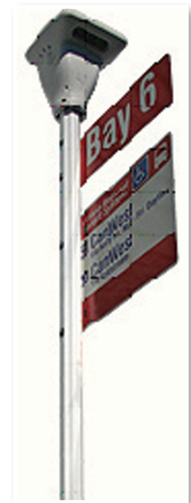
Example of a Solar Bus Stop Lighting System.
