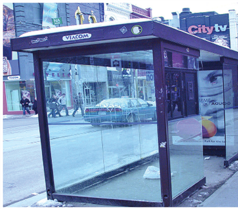
These two shelters in Toronto, Canada, open onto the sidewalk to provide protection from snow or water splashed by moving cars. The shelter is enclosed except for the entranceway to protect against inclement weather. Source: SUNY Buffalo
