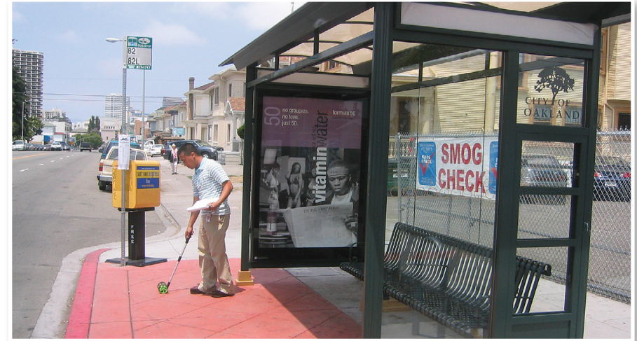
A transit agency official measures the distance between the edge of the shelter and the curb, using a measuring wheel, to determine if enough clearance is available for wheelchair users to board and alight the bus. Source: Nelson\Nygaard Consulting Associates
