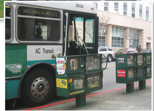
This stop in Berkeley, California does not have adequate clearance to deploy a wheelchair ramp. Additionally, the stop lacks identity, being indiscernible from a newspaper vending machine area. Source: Nelson\Nygaard Consulting Associates
