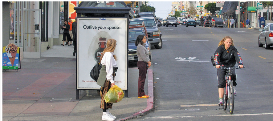
A bus bulb in San Francisco, California. The bus stop area is extended into the parking lane and incorporates a shelter that does not impede the pedestrian right of way. The bulb allows the bus driver to pull up flush to the curb to facilitate the boarding and alighting of passengers. Source: Nelson\Nygaard Consulting Associates
