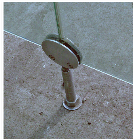
The glass panels of this bus shelter are raised above the ground to accommodate cleaning but not so high as to create a problem for people who use white cane. Picture taken in Toronto, Canada. Source: SUNY Buffalo
