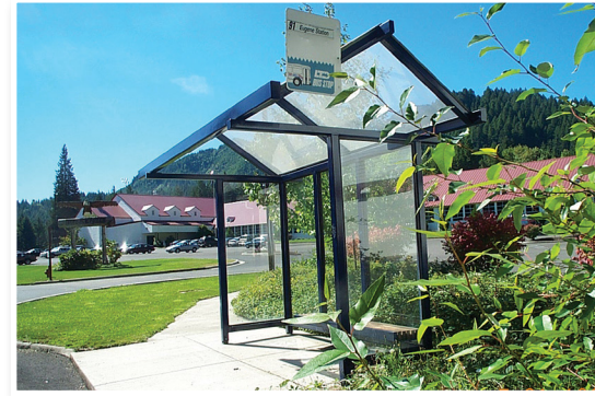
An accessible path is provided to and from the stop, linking the stop to the surrounding land uses in Eugene, Oregon. Source: G. Araki
