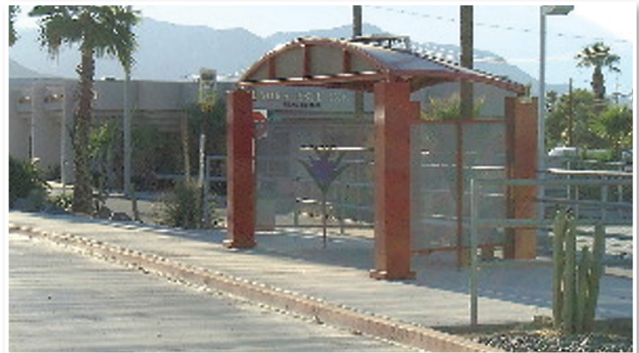
This shelter in Palm Springs, California allows air to circulate. The panels are constructed of perforated metal to allow airflow while maintaining good visibility of the surrounding area. Source: Robert Perrone Consulting
