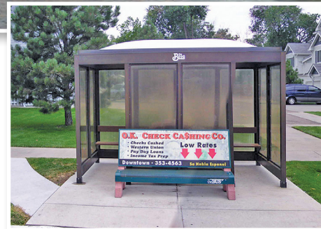
The exterior bench at a stop in Greeley, Colorado is poorly placed, obstructing access to the boarding and alighting area and into the shelter. The stop would otherwise be accessible.
