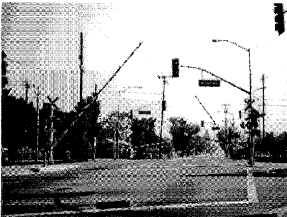
Exhibit 1 Typical quad gate at-grade crossing
