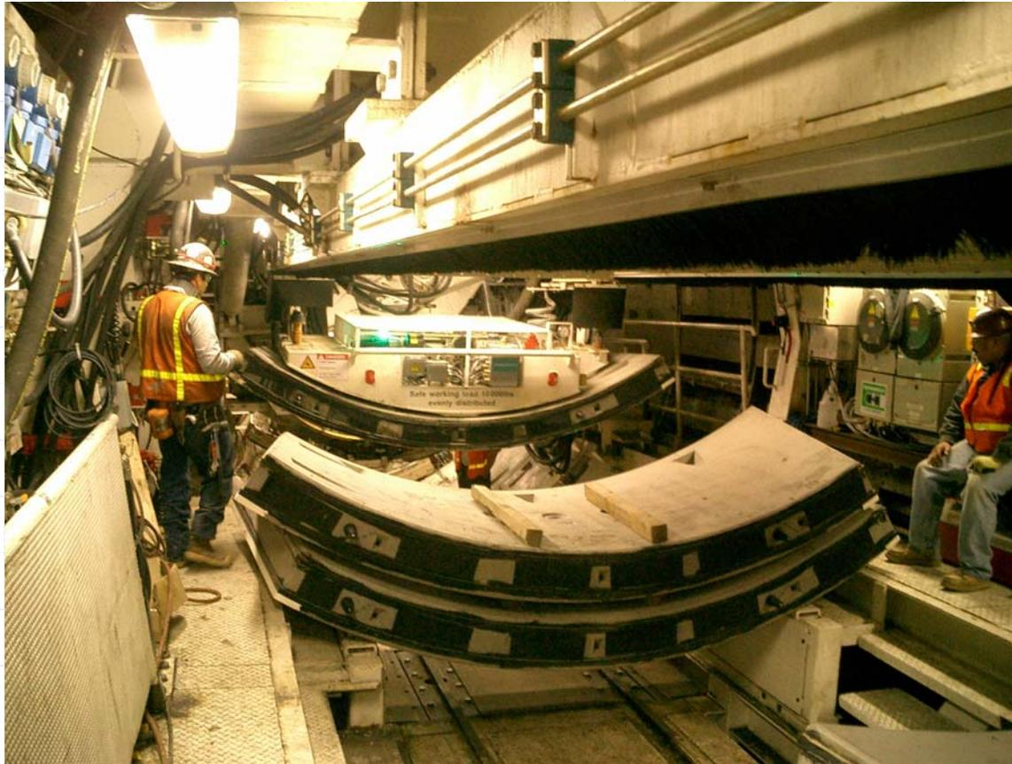
Installation of precast tunnel segments.
