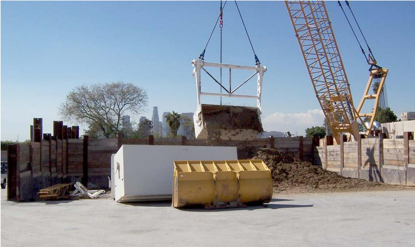
Tunnel mucking operations at the ground surface.
