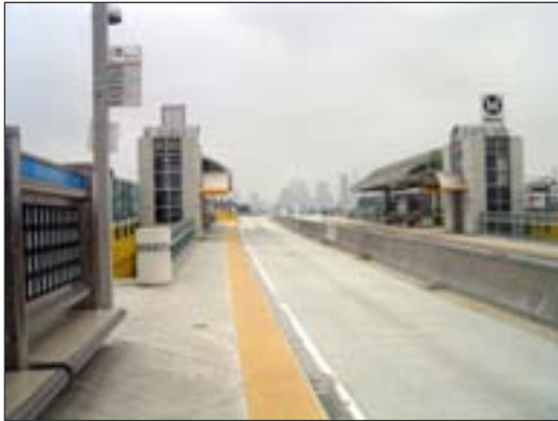
Harborway Transit Center at freeway grade
