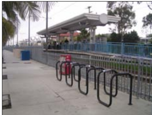
Bike racks at Willow Station
