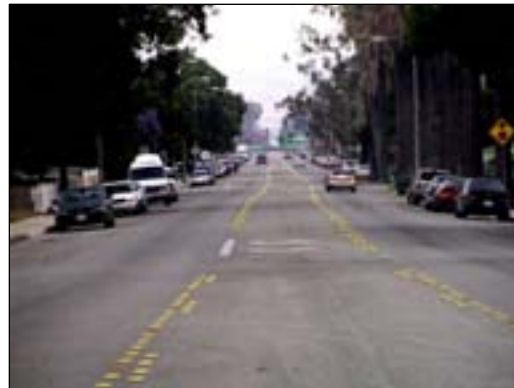
Alvarado Street and Park Avenue looking southbound
