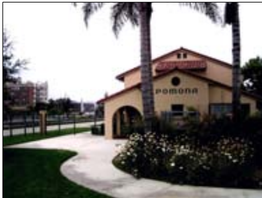
Pomona Metrolink Station
