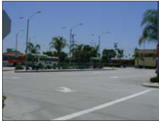
Inglewood Bus Center bus turnaround
