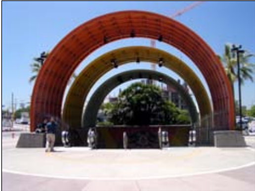
North Hollywood Metro Red Line station
