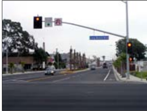
Spring Street at Long Beach Boulevard
