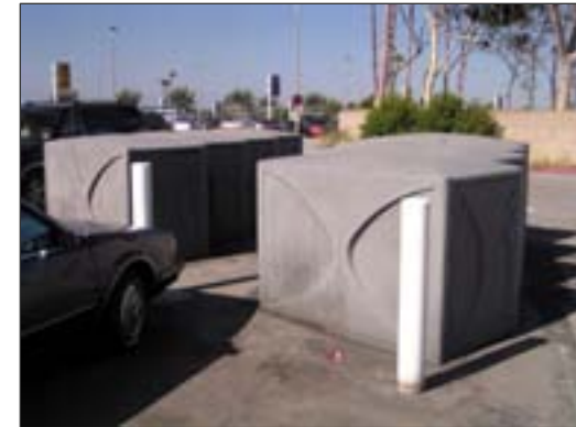
Lockers at Bus Center
