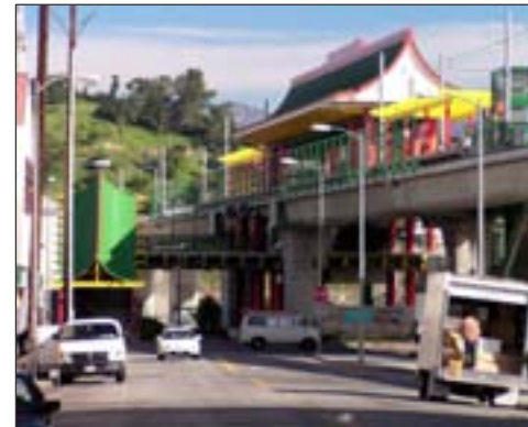
Spring Street facing north towards station
