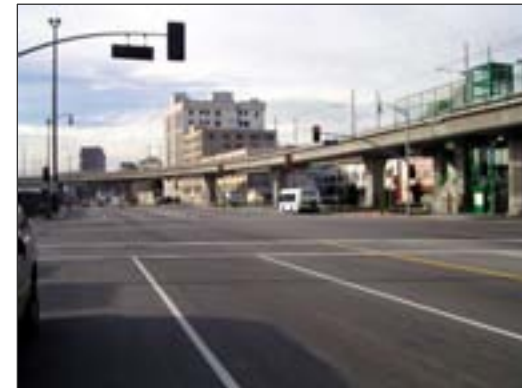
Alameda Street facing south across College Avenue
