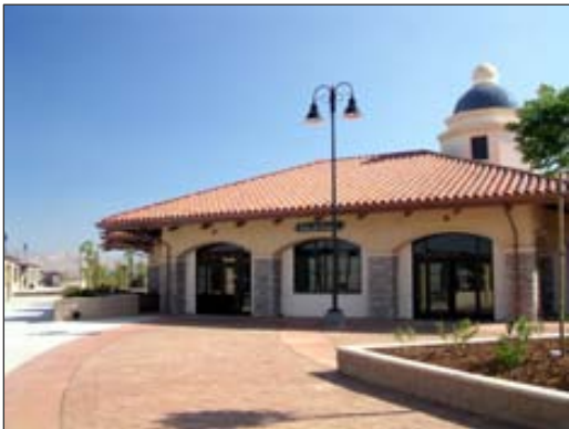
Palmdale Transportation Center
