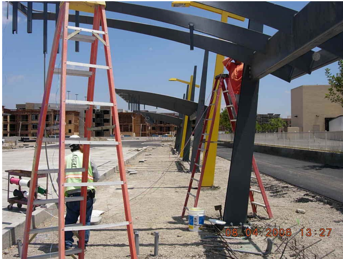
Wire pulling at eastbound platform
