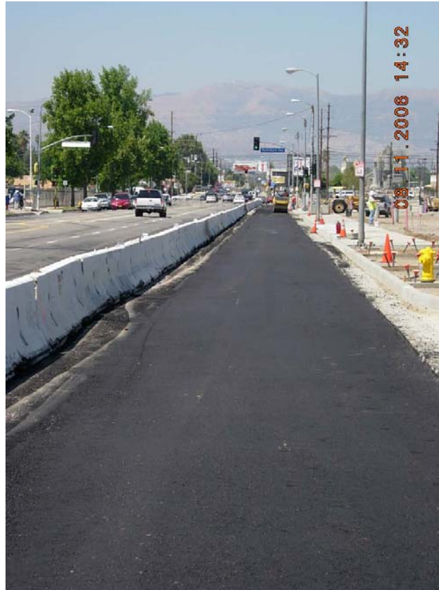
Paving of widened portion of Canoga Avenue looking north
