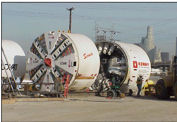
Figure 4-1 ECIS Project EPB Machine Being Assembled
