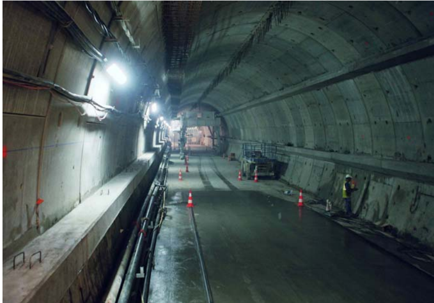
Figure 4-5 Precast Segmental lining for A-86 Tunnel, France
