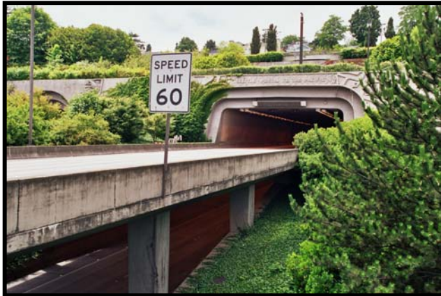
Figure 2-4 East Portal – Shows Approach Structure and Reversible Lanes Below
