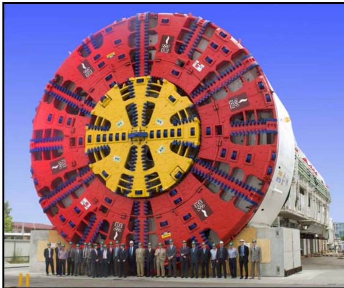
Figure ES-2 Tunnel Boring Machine – Madrid, Spain
