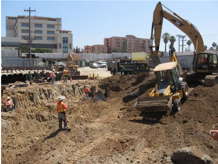
Excavation of Station Entrance
