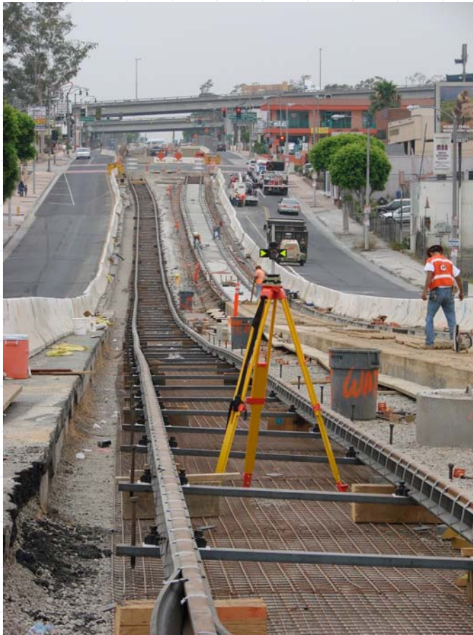
Installation of trackwork and Overhead Contact System catenary wire pole foundations along 3 rd Street.
