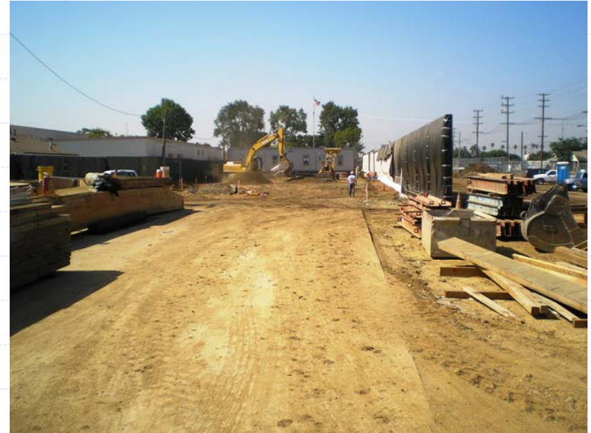
LAUSD's contractor performing site work
