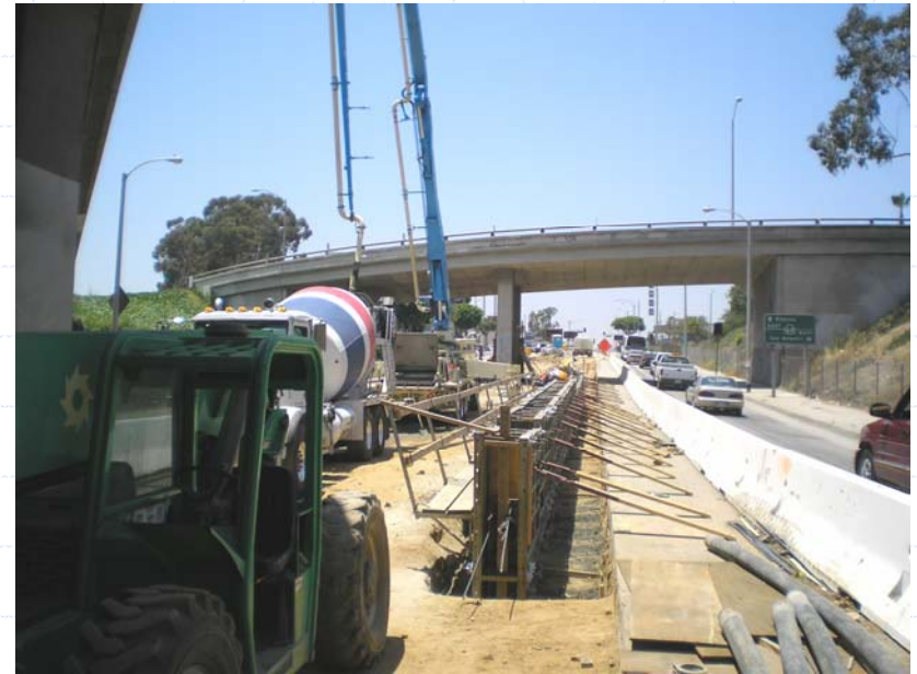
U-Channel on 3 rd Street between Marianna and Downey
