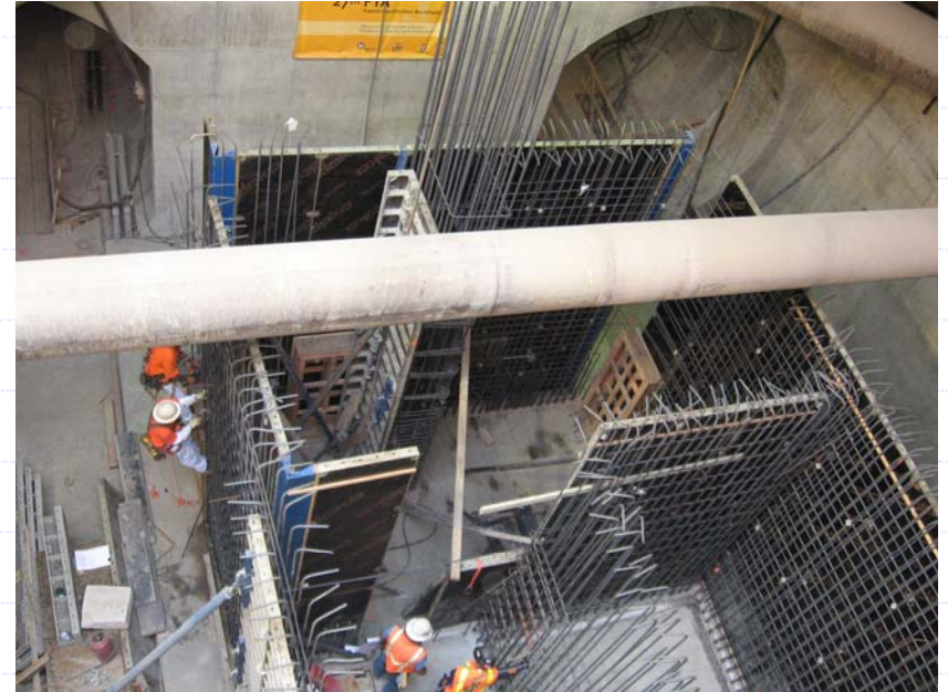
Interior Rooms Below Mezzanine Level
