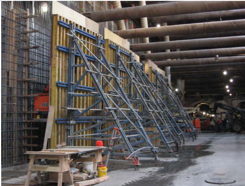
Formwork is placed for the concrete wall pour
