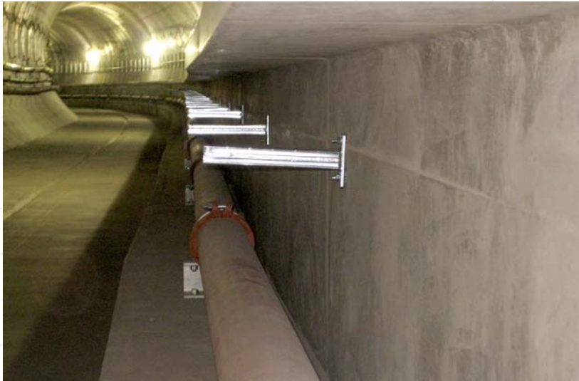
Tunnel invert slab and walkway
