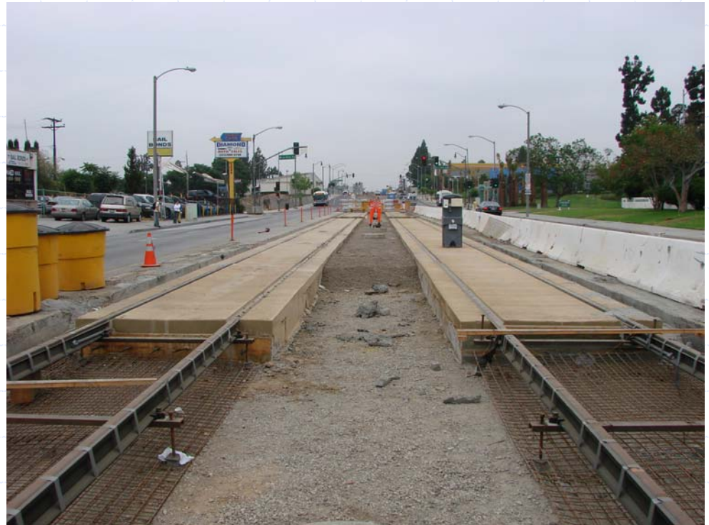
Installation of trackwork and Overhead Contact System catenary wire pole foundations along 3 rd Street.
