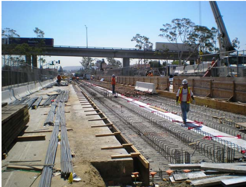
I-710 Freeway Bridge on 3 rd Street near Ford
