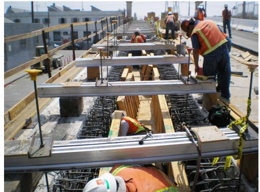
Steel reinforcement bars are being installed for the girder strengthening
