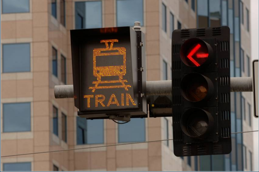
LED sign indicate approach of trains
