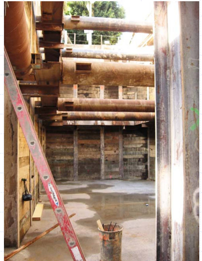
Soto Station area of future emergency exit at mezzanine level.
