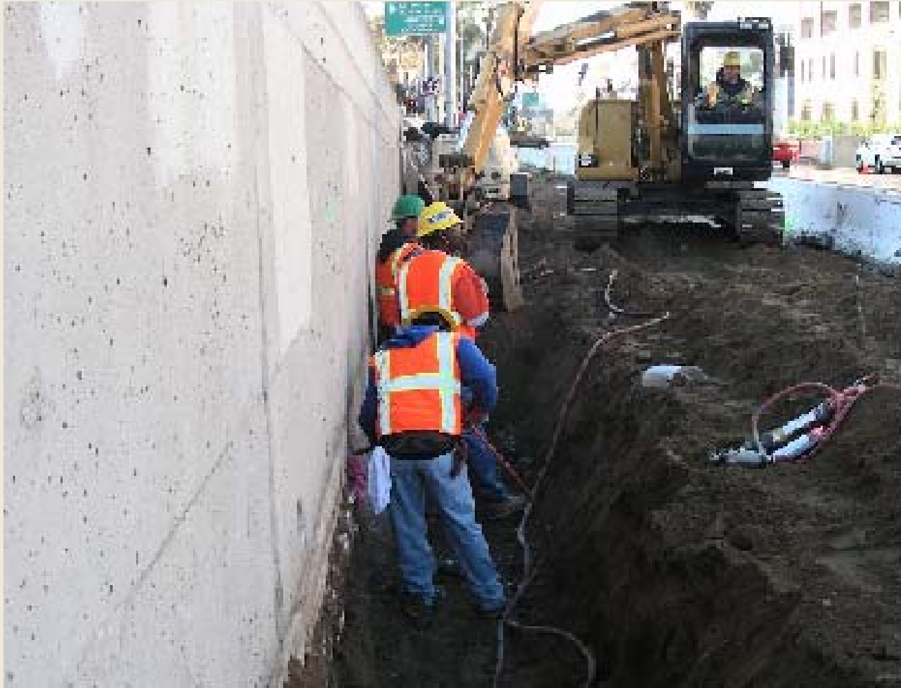
Excavation for Storm Drain on Flower
