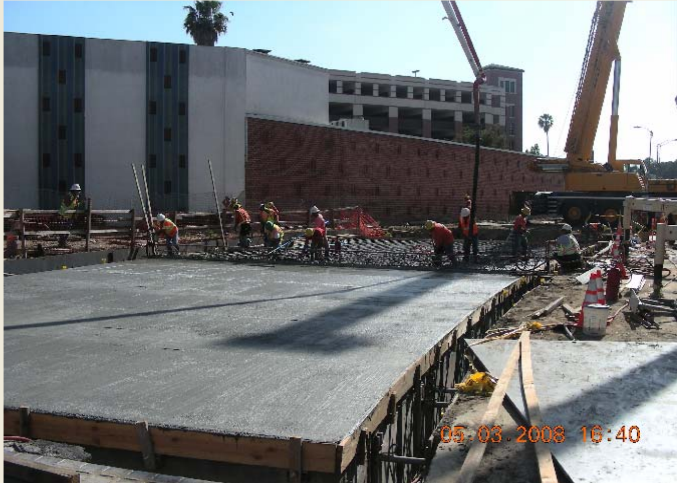
Concrete Deck over Girders at Exposition and Flower
