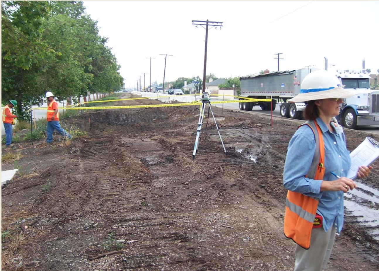
Soil Removal in Segment B
