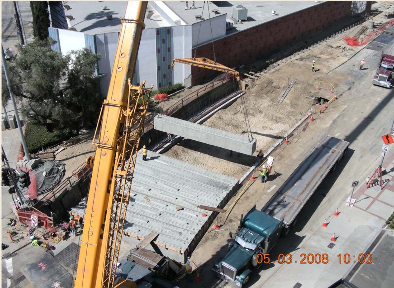
Installation of Box Girders along Exposition and Flower
