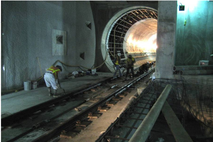
Trackwork installation at westbound tunnel interface at 1 st /Soto underground station.
