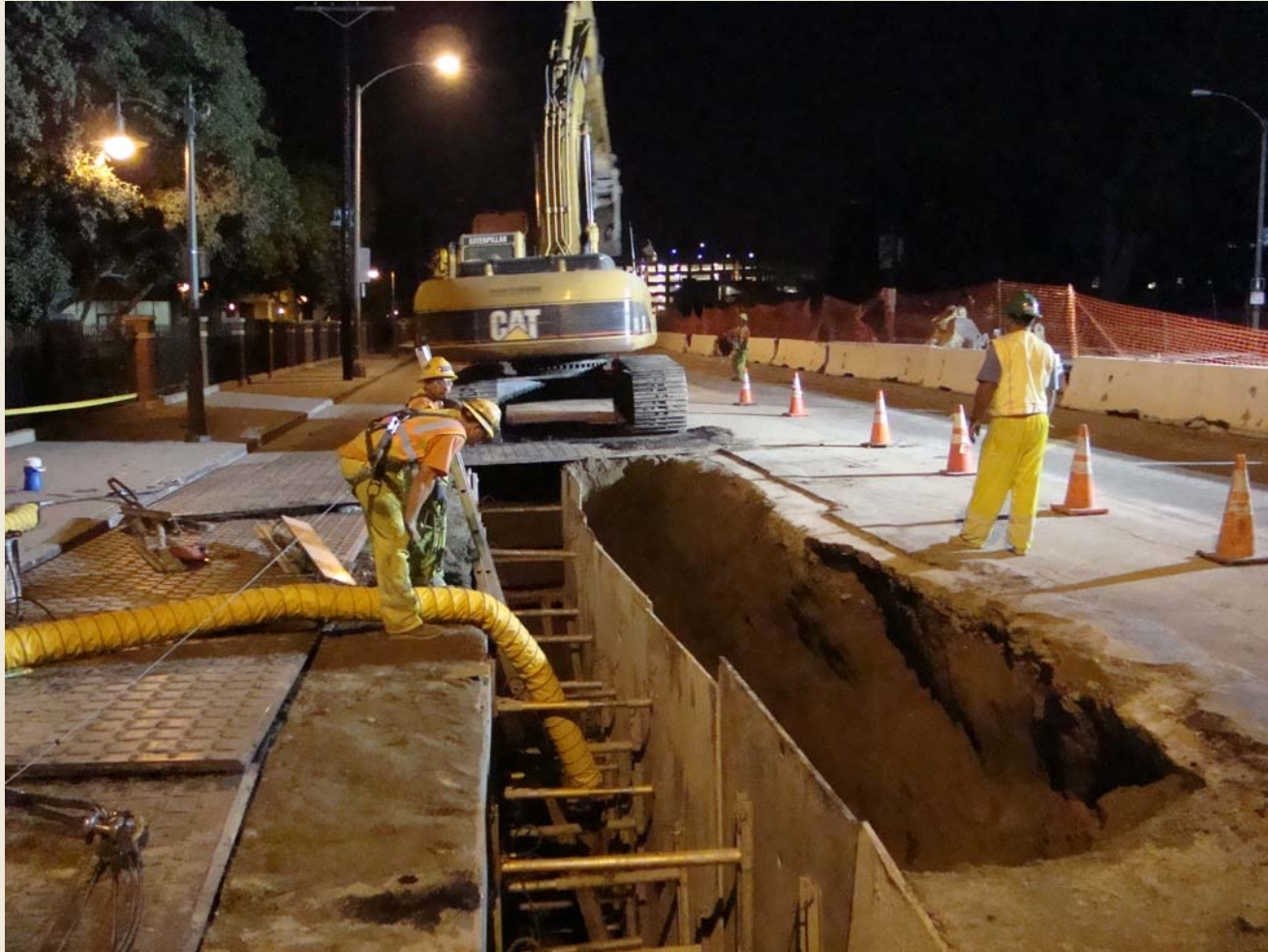
Installation of VCP Sewer Line at Exposition Blvd. and Watt Way
