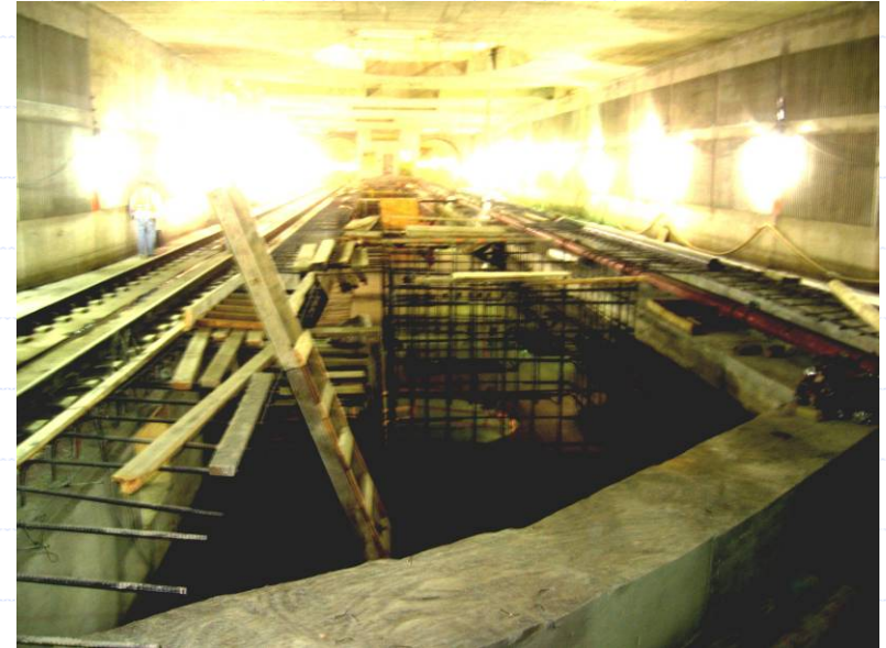
Steel reinforcement installation for concrete structures at the train platform level.
