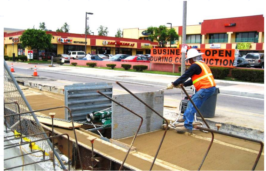
Systems installation work progresses at the Pomona/Atlantic Station.
