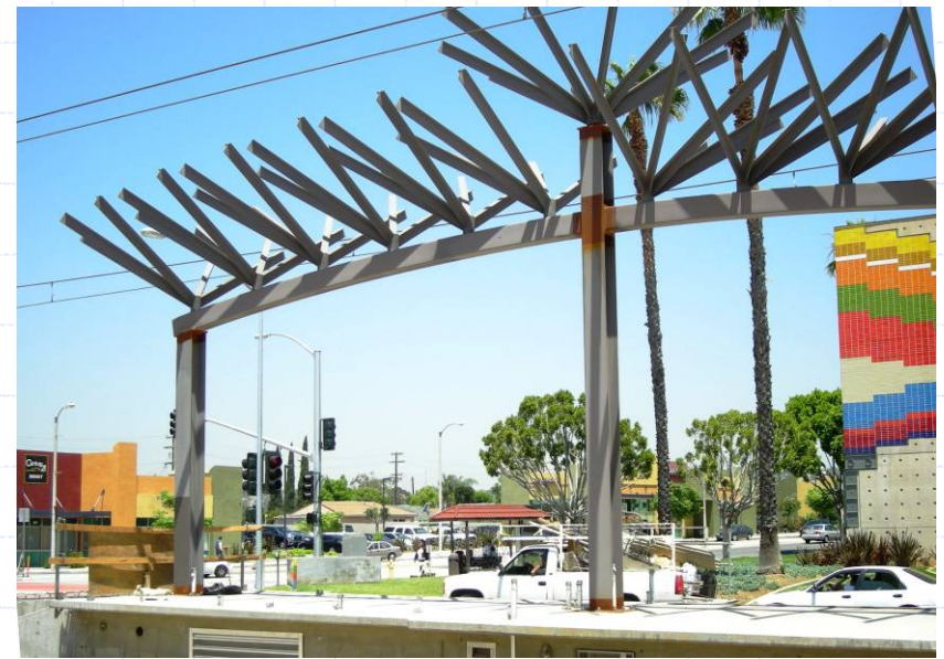
3 rd /Mednik - East Los Angeles Civic Center Station
