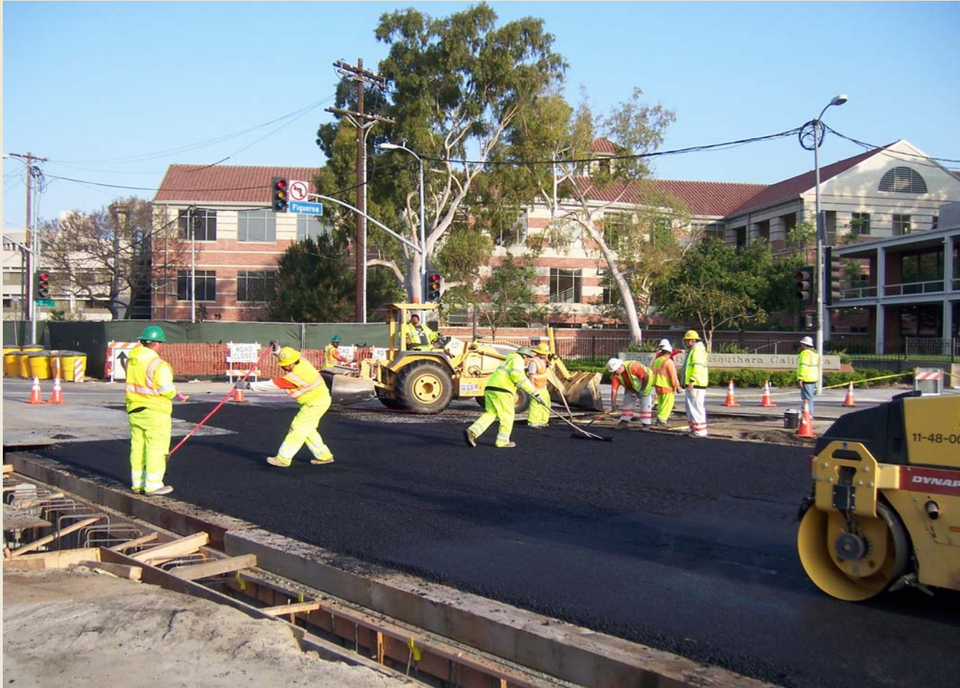
Temporary Pavement in Front of USC
