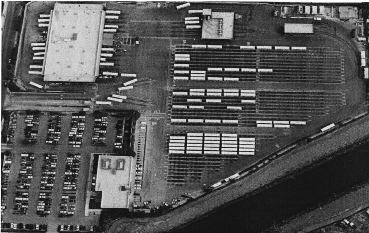
Division 18 (Carson) – Although Landlocked, Offers Potential to Expand with a Second Story Deck
