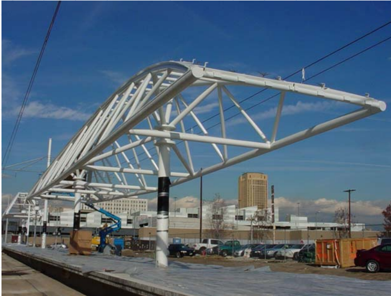
Little Tokyo/Arts District Station - Northeast corner of 1st/Alameda.
