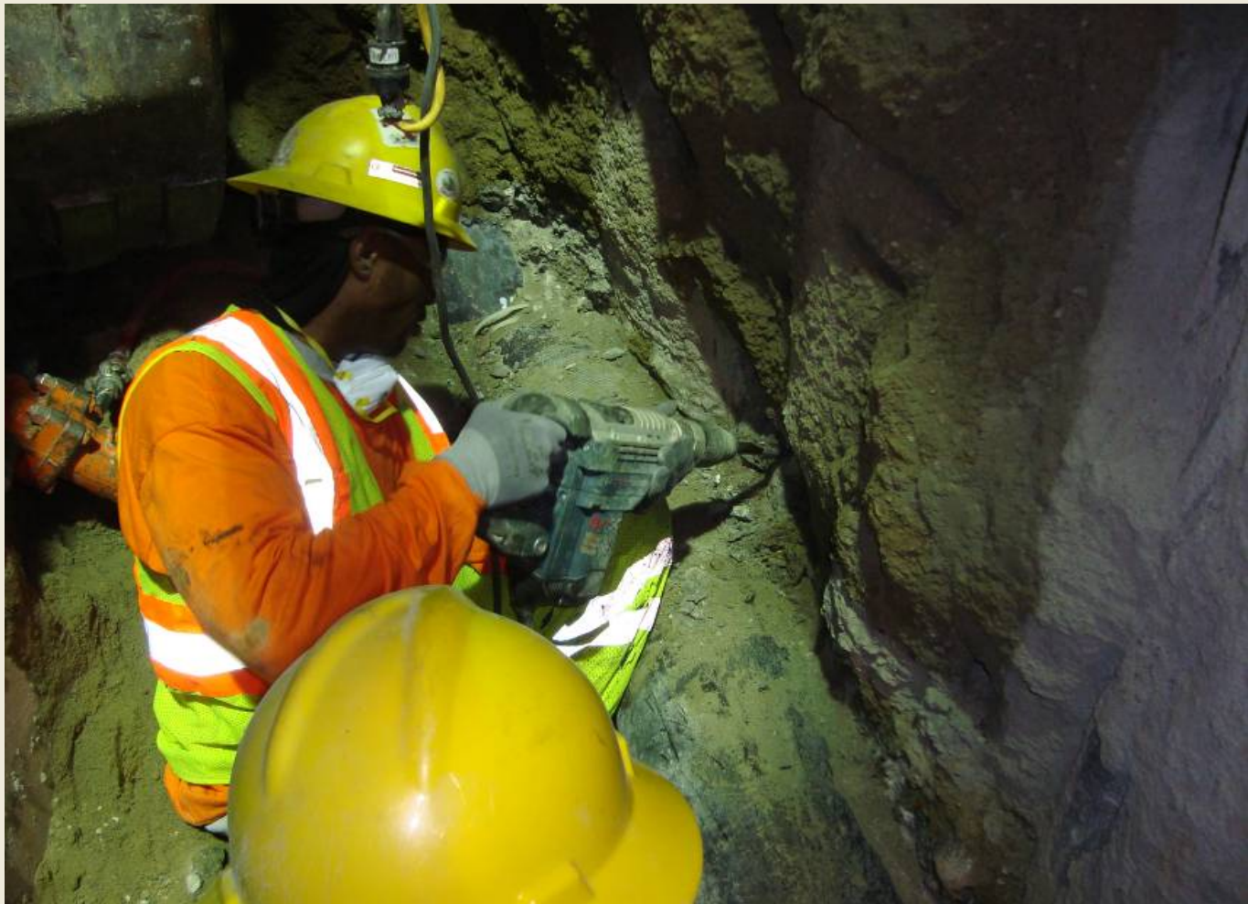
Sewer repair work at Flower and Exposition
