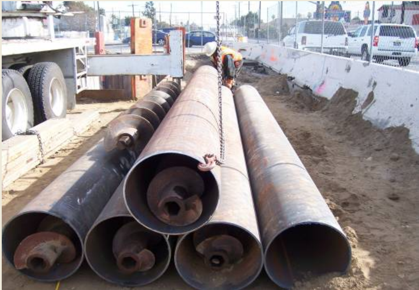
Preparation for jacking operation at Exposition and Western
