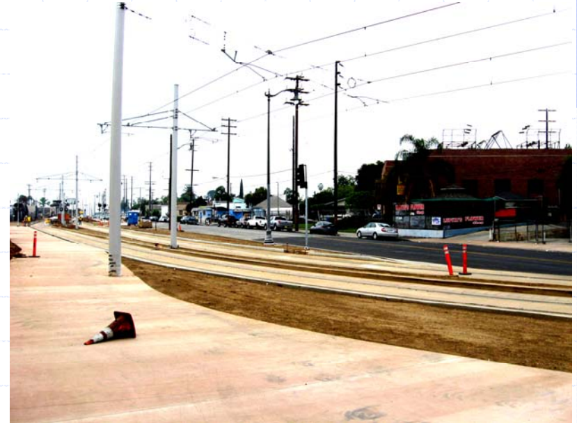
Indiana Street view south towards 3 rd Street.
