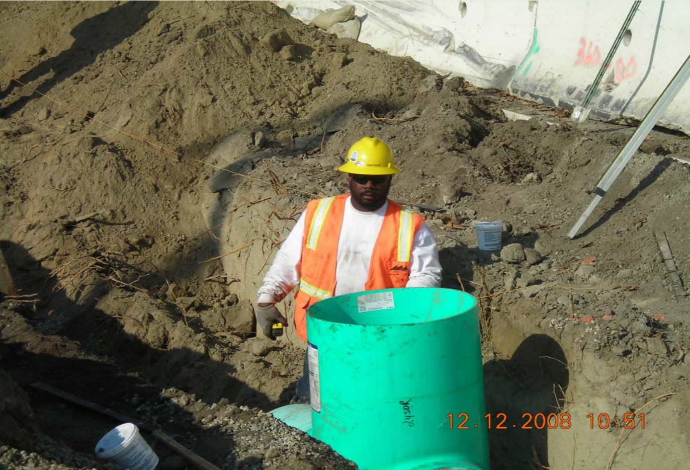
Installation of track drain along the ROW
