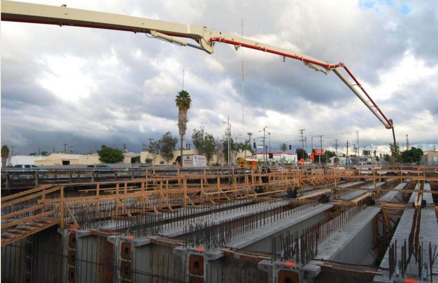
National Bridge Girder Closure Pours
