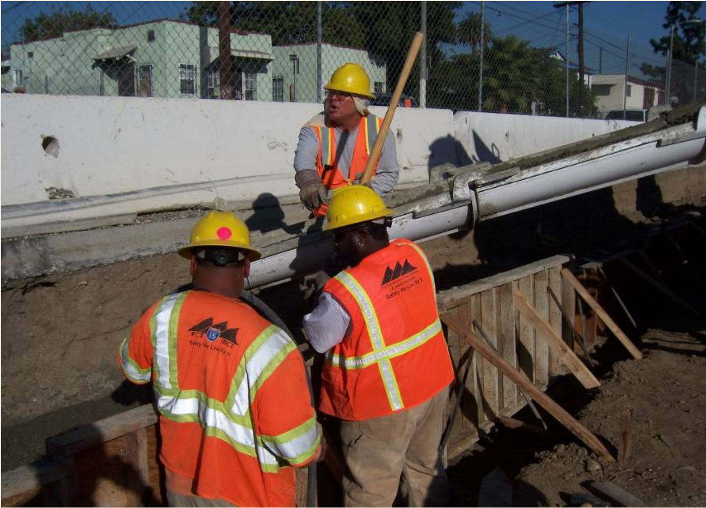
Concrete encasement of 18" PVC track drain
