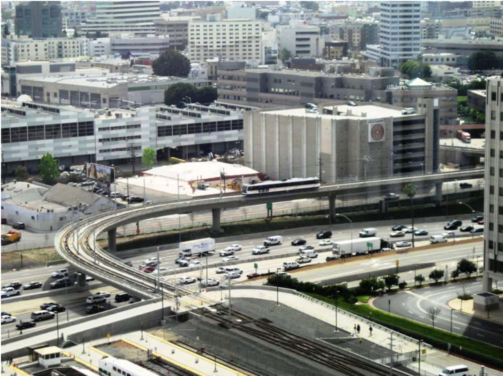
Light Rail Vehicle on aerial guideway structure crossing the 101 Freeway at Union Station.
