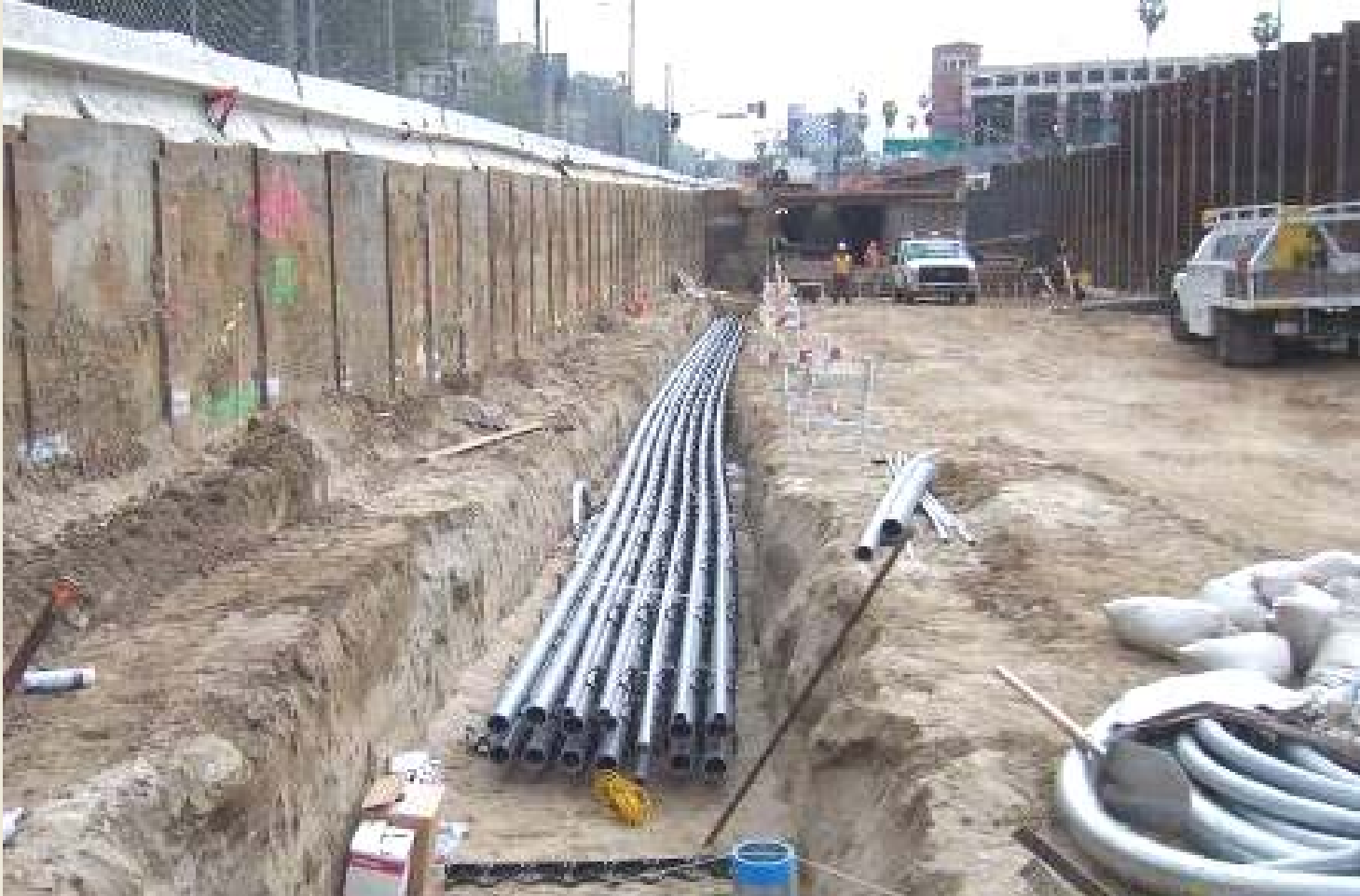
Conduit Installation at Exposition Portal of Trench Structure
