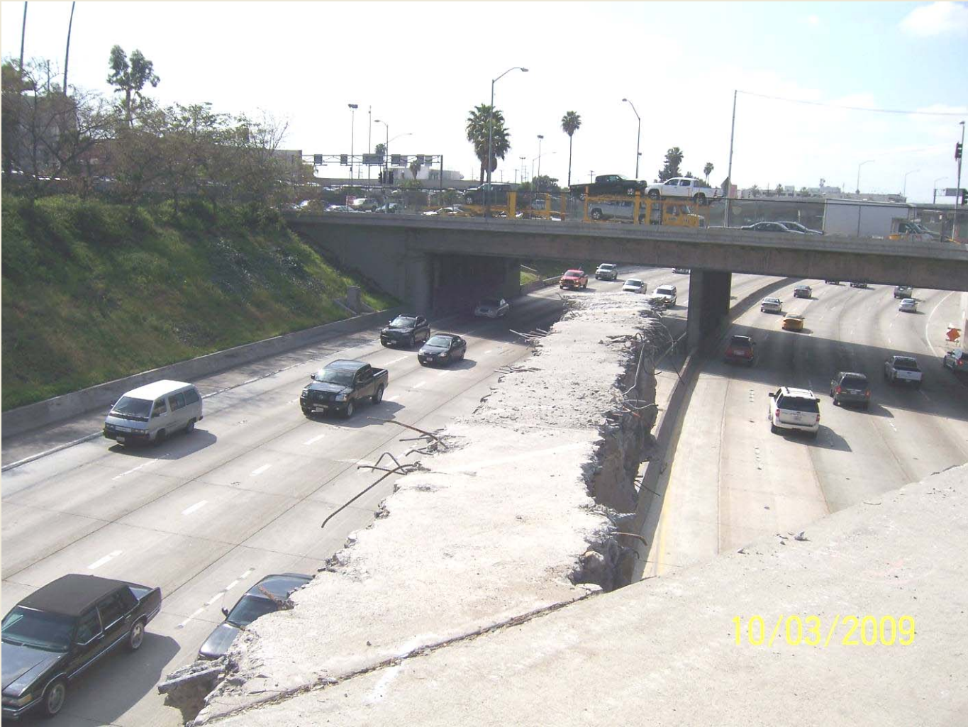
Flower Street Overcrossing Above I-110 Freeway After Completion of Girder Demolition
