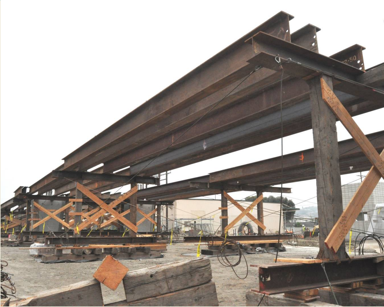
Installation of Falsework at La Cienega Overcrossing
