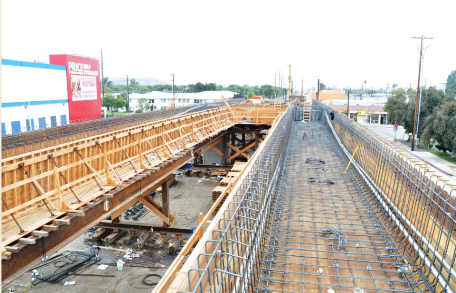
Installation of Stem Walls and Soffits at La Brea Overcrossing Structure
