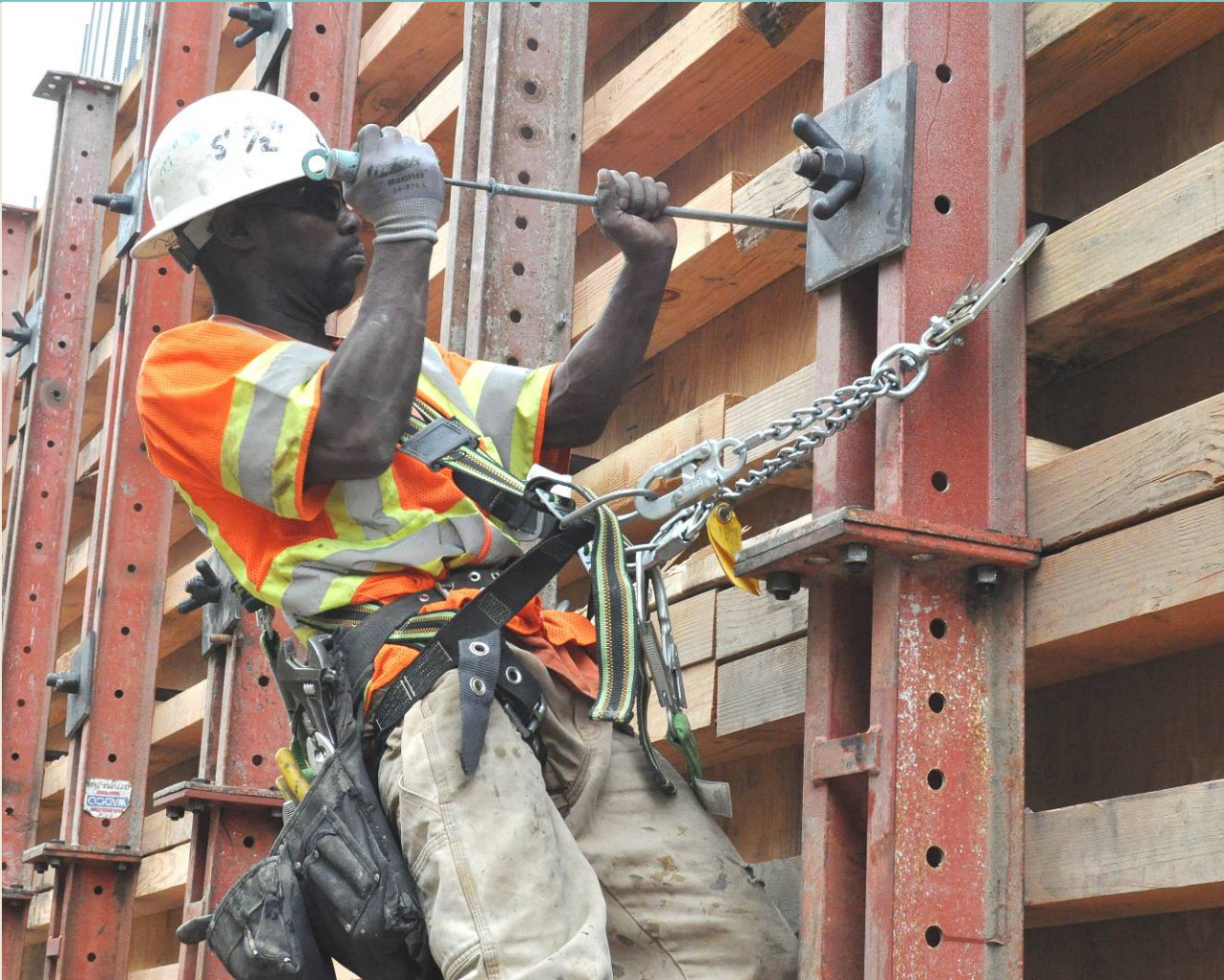
Forming of the U-Section at the Grade Separation Trench Structure
